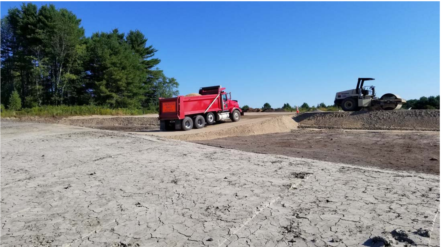
Access ramps from the compost pad area were temporarily built for truck access to the landfill.
