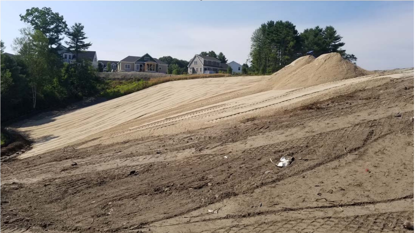
Placing the gas vent sand over the southwest slope of the landfill.
