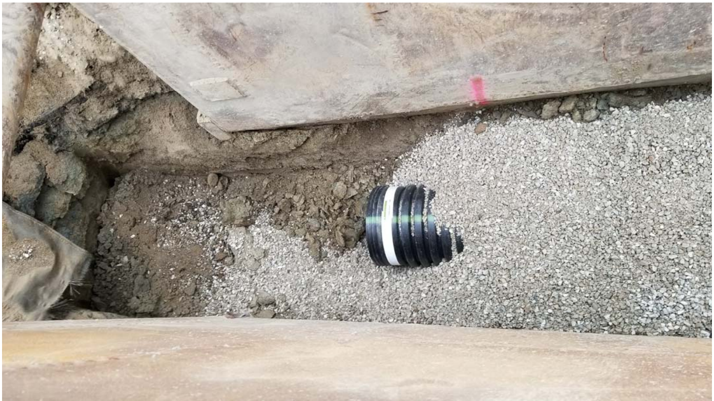
Backfilling around stormdrain
