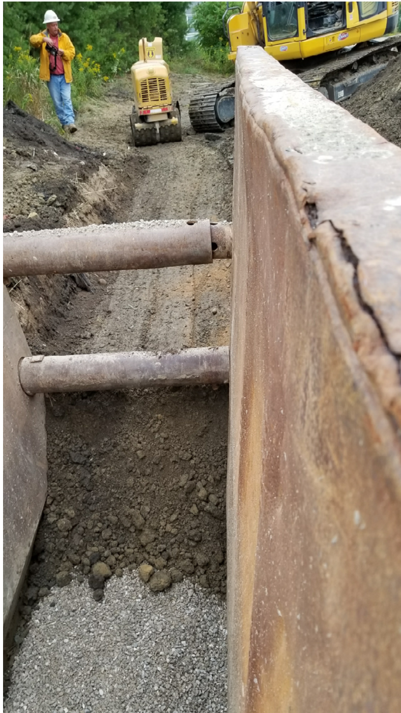
Compacting the backfill over the drainage stone.
