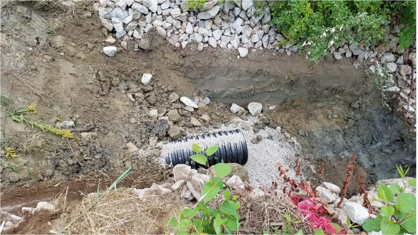
Outlet in place behind salt shed.
