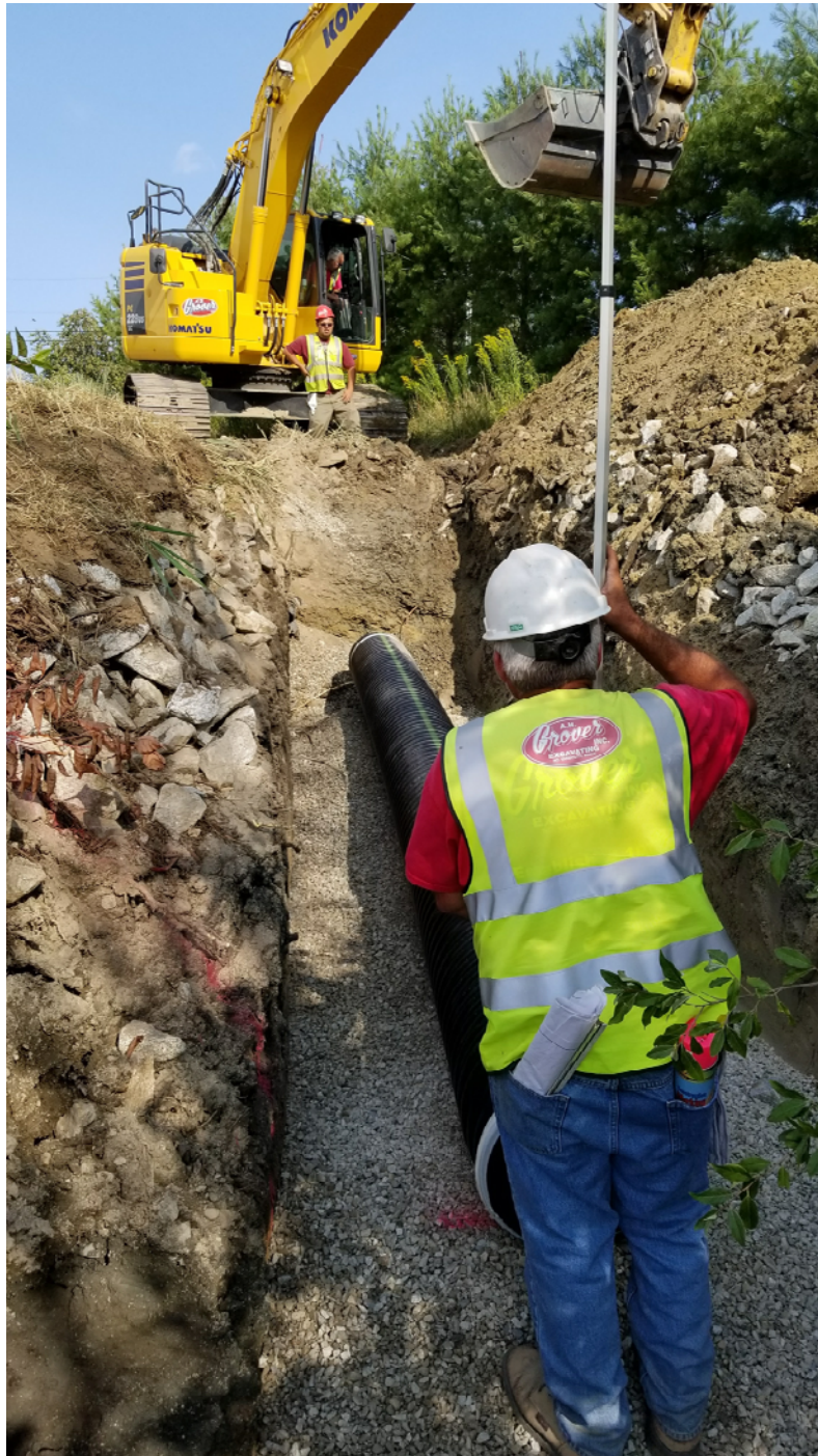
Placing first section of stormdrain behind the salt shed.
