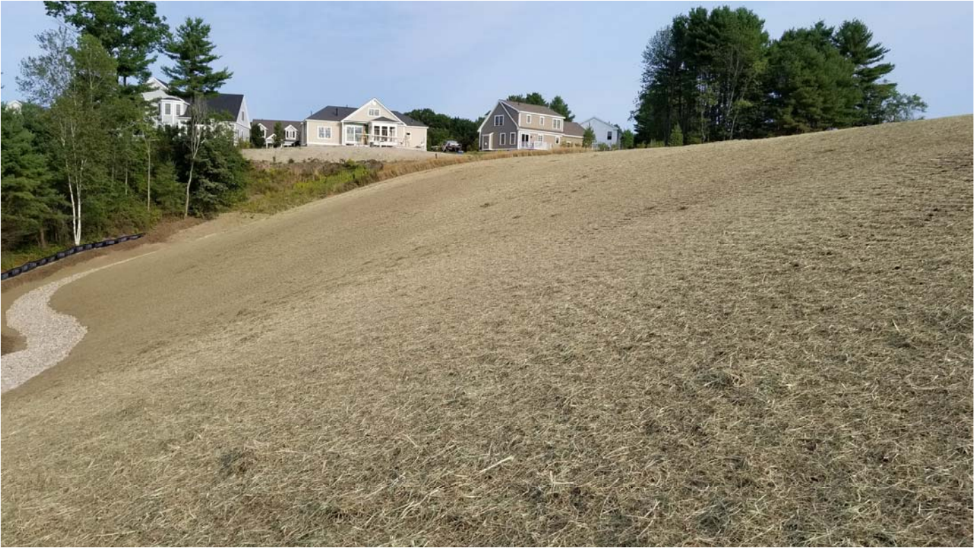
Mulch over the seeded topsoil.
