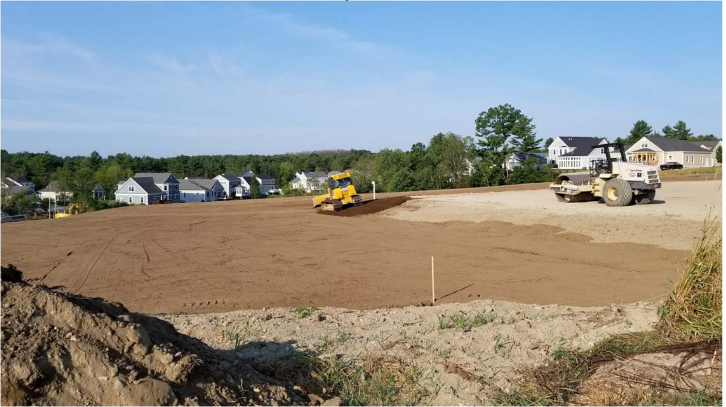
Placing topsoil along the edge of the compost pad.
