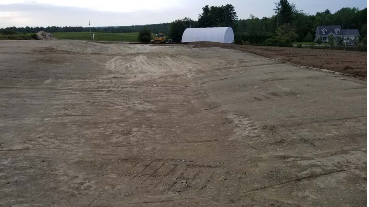
Finished the barrier soil and began placing the topsoil on the northeast corner of the landfill.
