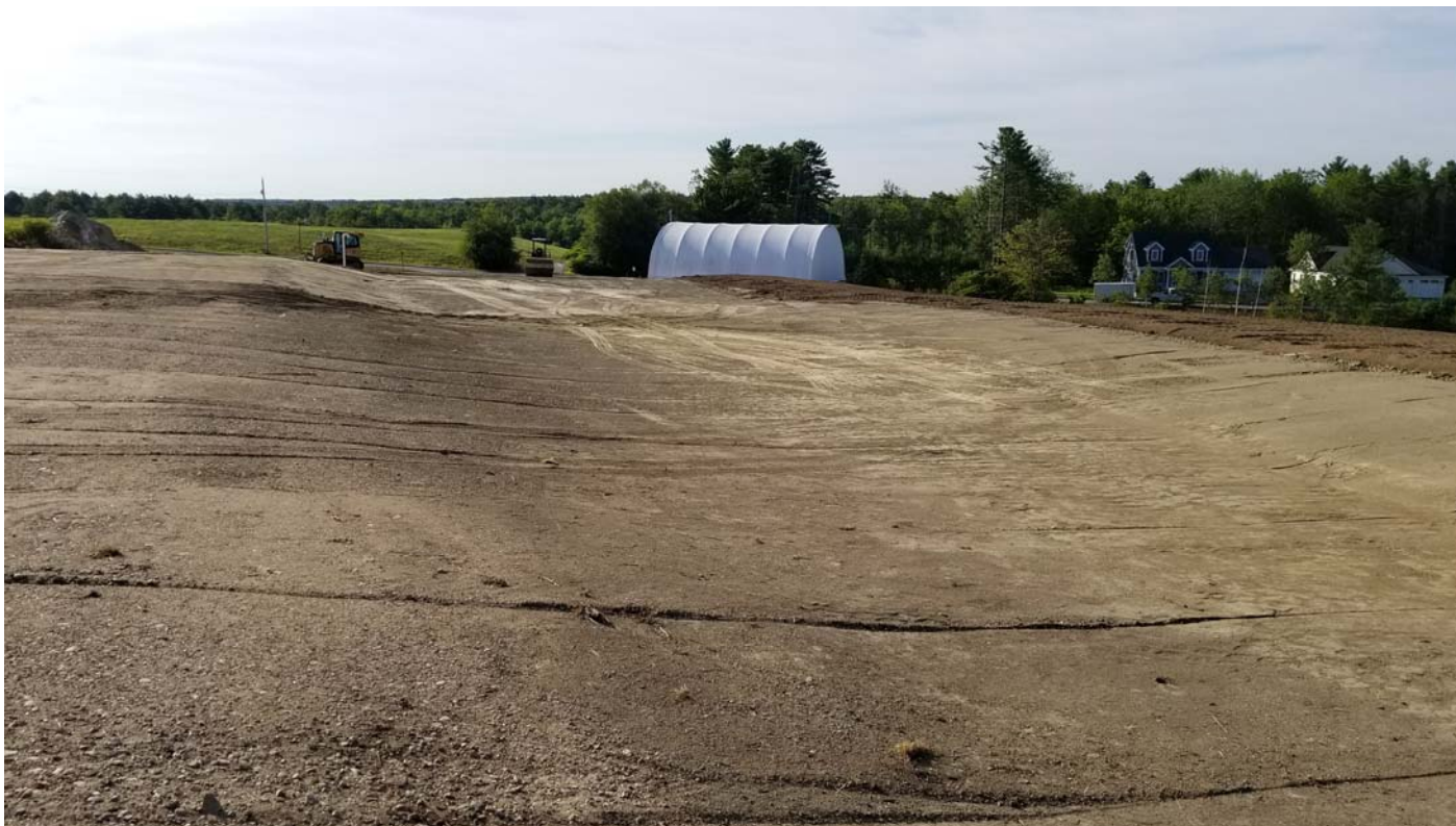
Placed 6" of gas vent sand, 18" of barrier soil, and then common borrow over the gas vent pipe.
