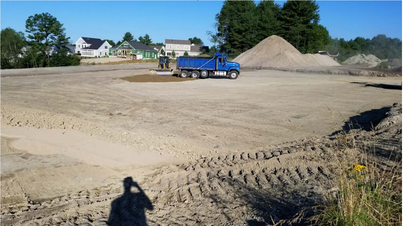
Placing the last lift of barrier soil over the northeast corner of the compost pad area.
