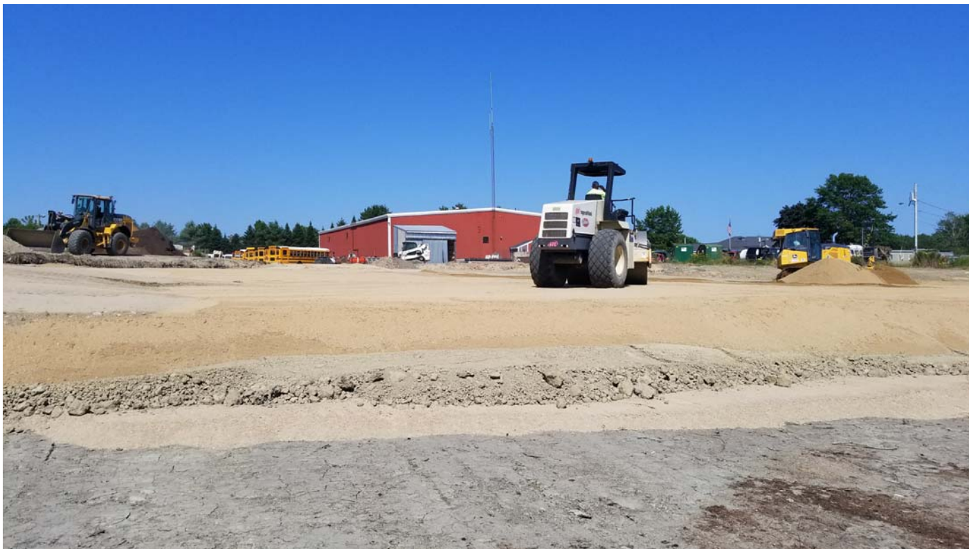
From the south side of the compost pad looking north. Gas vent sand layer on the bottom, with clay and then common borrow on top.
