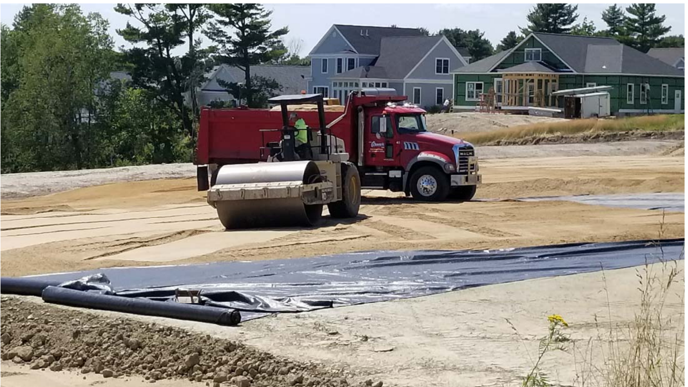
Compacting the first lift of common borrow with the geotextile stapled underneath.
