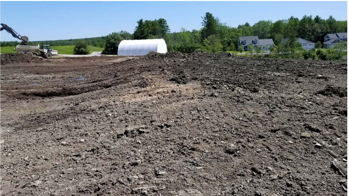
Filling behind the berm using the clean cut from the hole used to bury the larger woodwaste and dirty debris.
