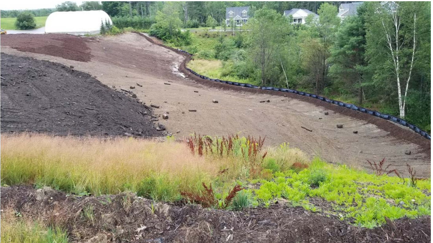
Placing the cut from the compost pad on the southwest slope of the landfill.
