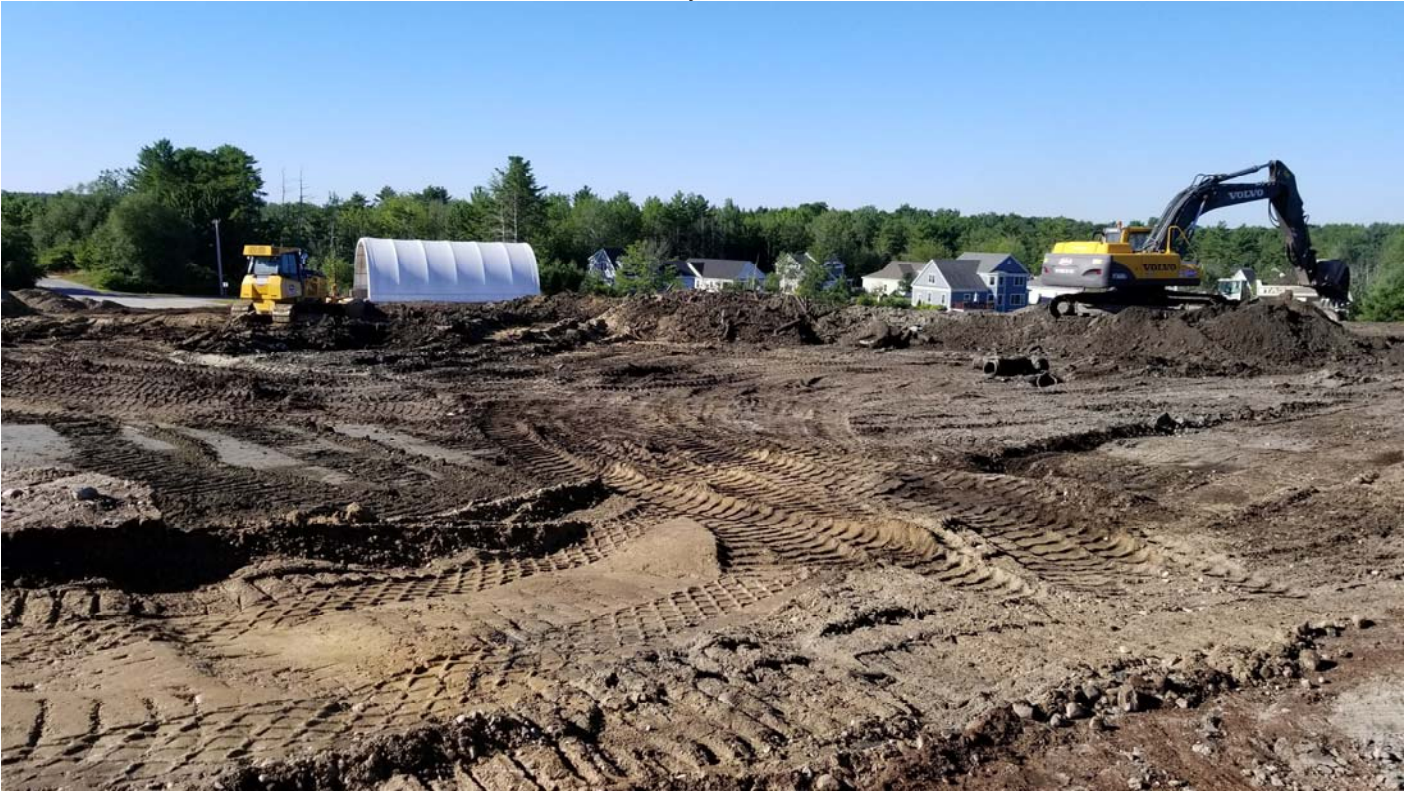
Removing the remainder of waste from under compost pad and preparing the subgrade.
