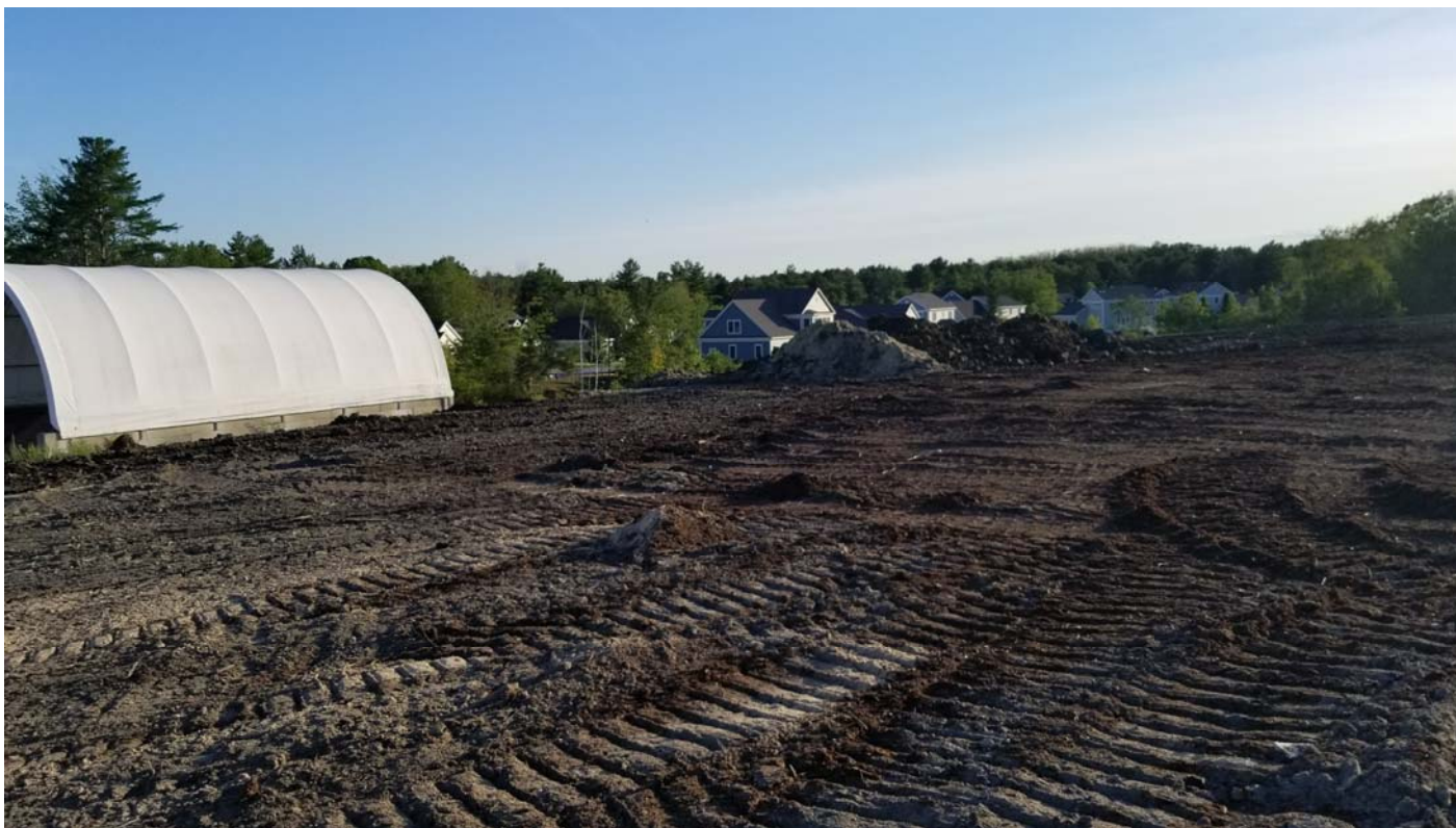
The final piles of fill at the end of the diversion berm. Subgrade finalized on the remainder of the site.
