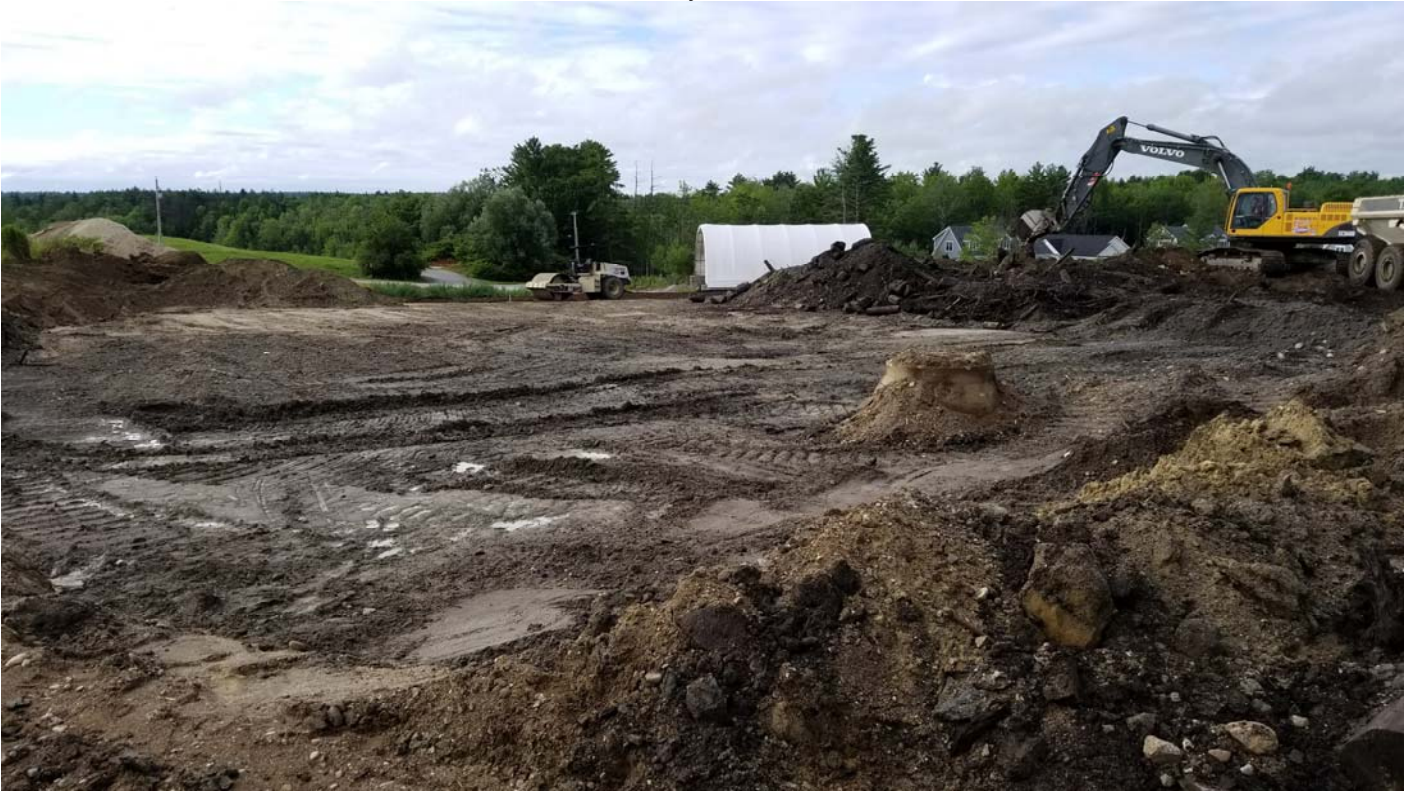
Removing waste from under compost pad and preparing the subgrade.
