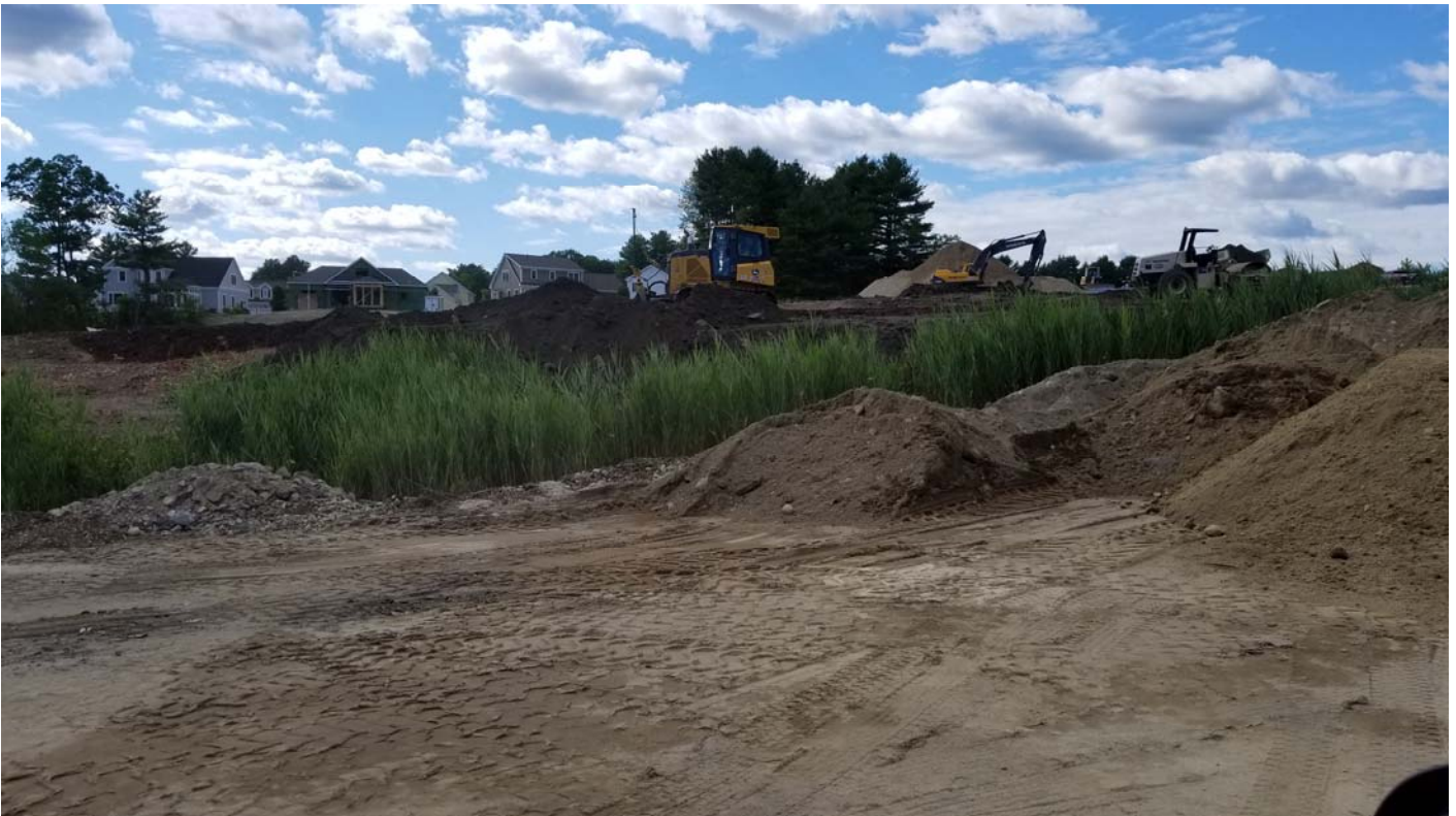
Placing the cut from the compost pad on the eastern slope of the landfill.
