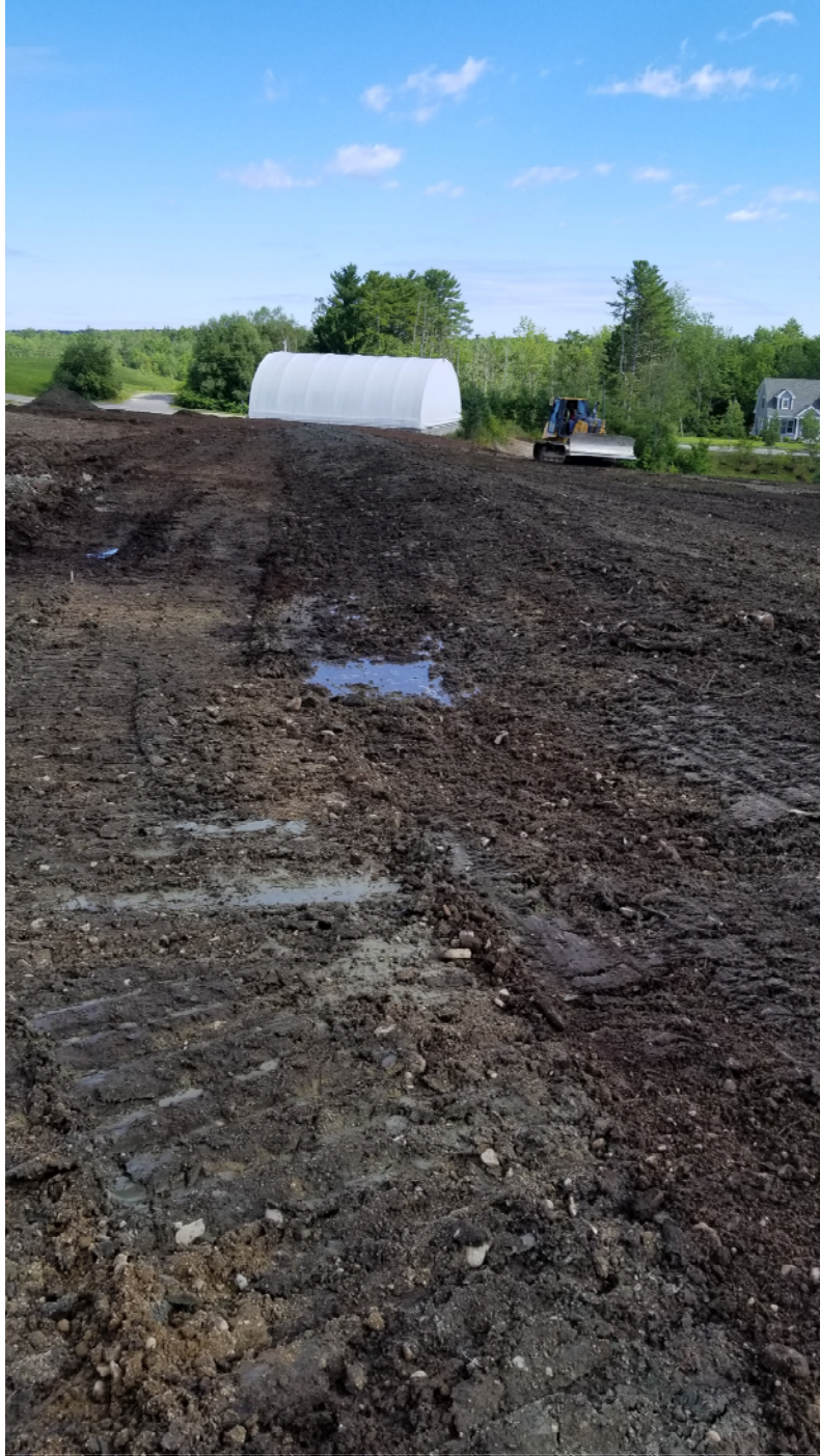
The diversion berm graded into the waste from the west side to the east.
