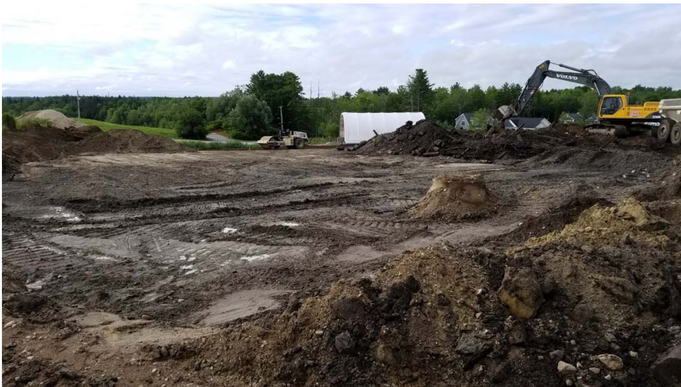
Pulling back the waste from under the compost pad.
