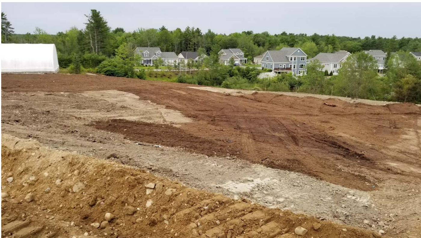
Once spread, the compost was rolled to minimize the impact to fill volume.
