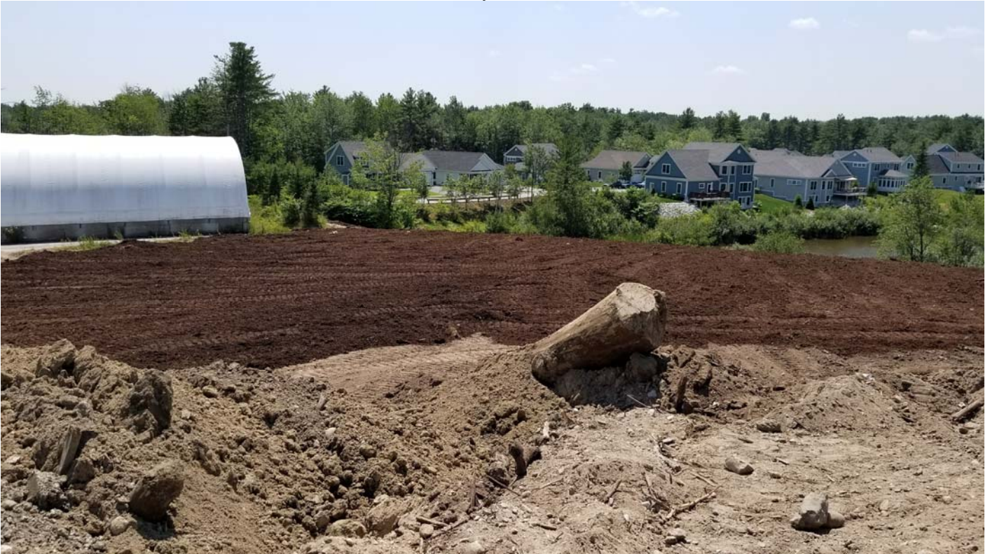
The compost piles left on site were spread across the top of slope.
