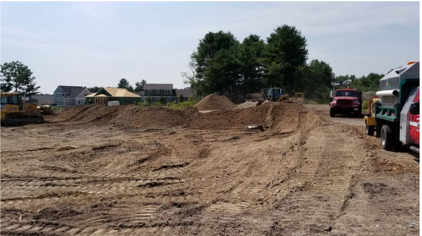
The existing gravel pad was scraped off and then stockpiled in the background.
