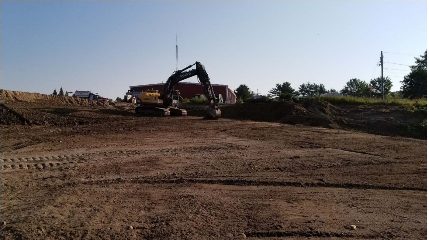
Fill excavated from east of the compost pad, placed at edge of slope, and pushed into place.
