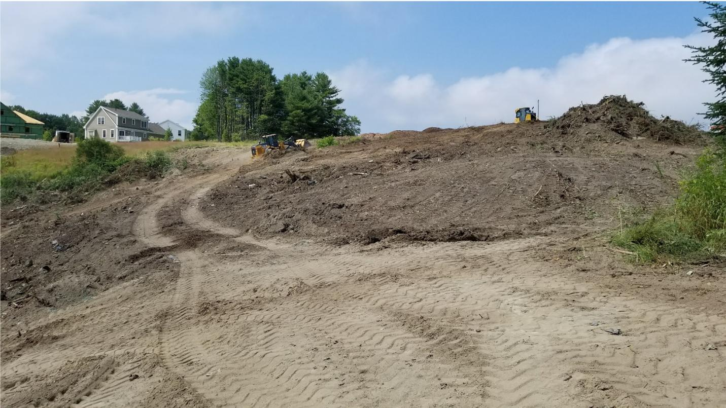
Clearing and grubbing inside clearing limits.
