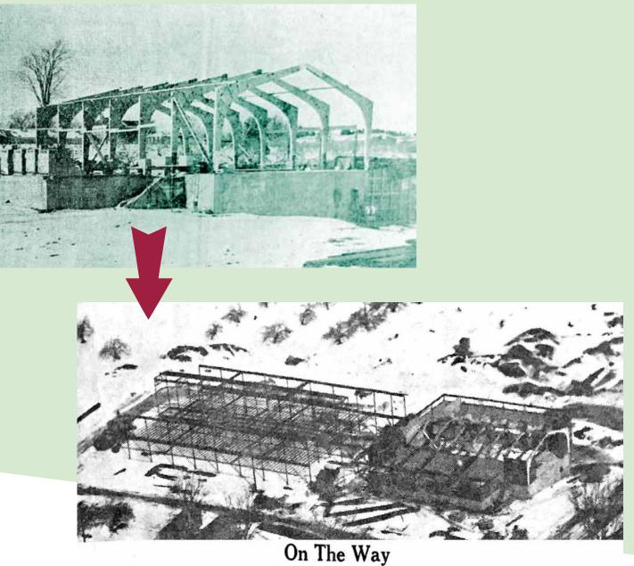
Beginning to take shape is the new Cumber- tive office section is in the right foreground. Beland elementary school on Tuttle Road there. The hind it are the arch-shaped frames of the multiframework at the left is for a two-story wing purpose room. The kitchen area will be behind the which will house 16 classrooms. The administra- multipurpose room. (By Staff Photographer Roberts)
