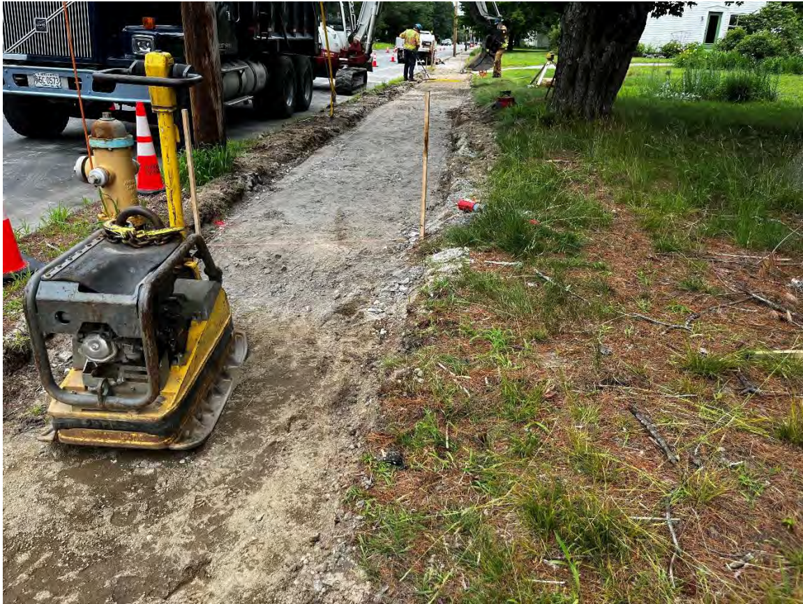
Photo 7 – Wacker Neuson Plate Compactor used for compaction efforts.
