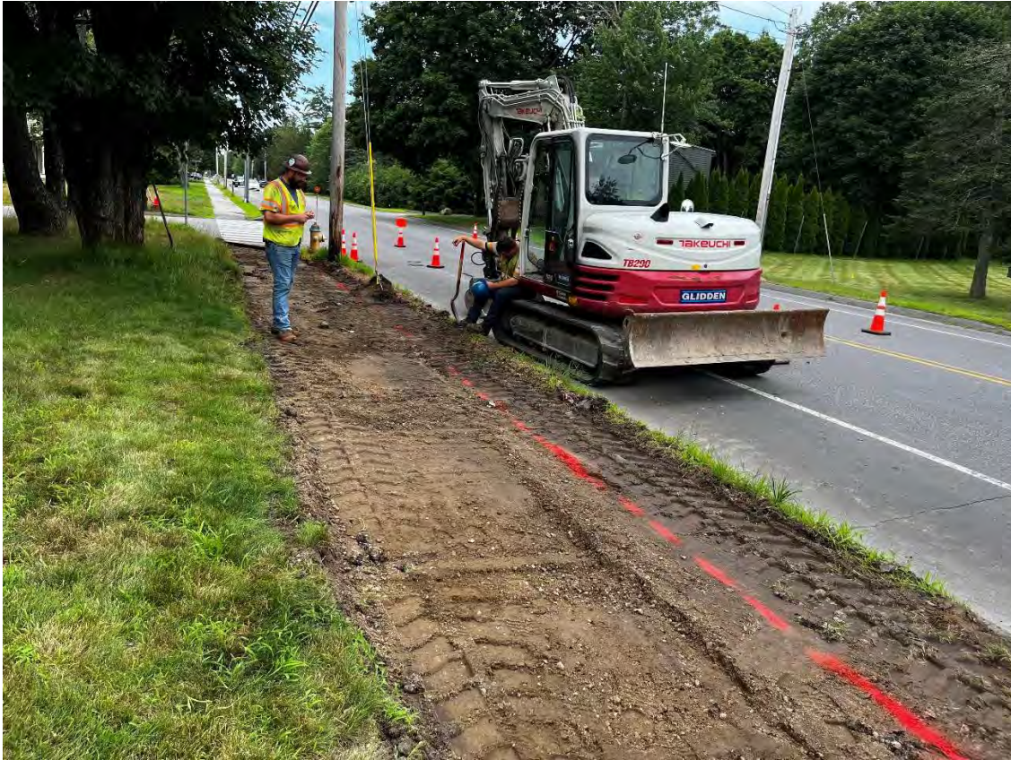
Photo 1 – Existing pavement removed to Hillcrest Drive.
