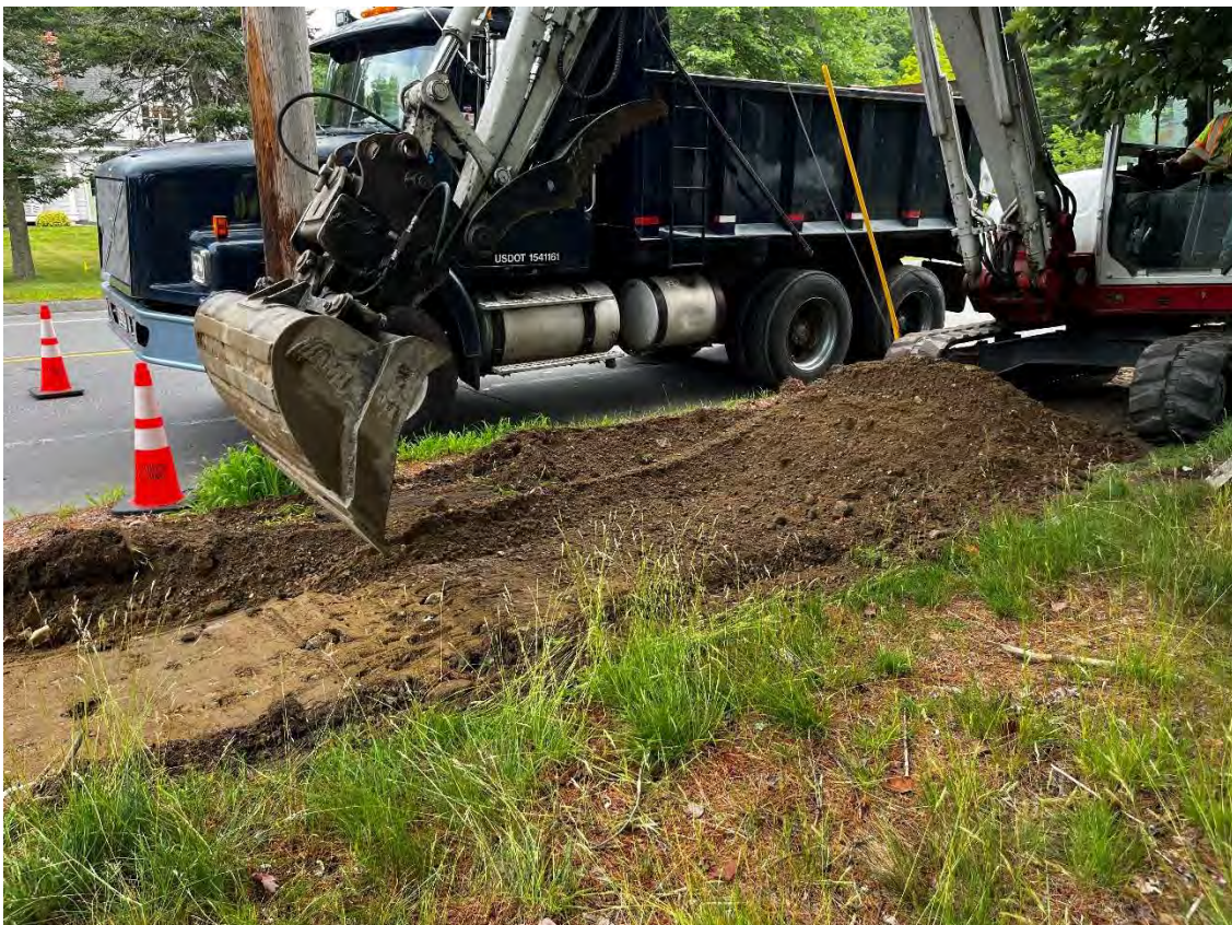
Photo 2 – Top 12" of existing gravels excavated.
