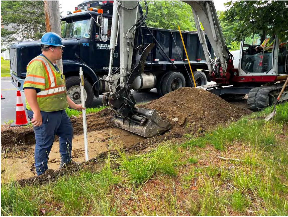
Photo 3 – Crew member holding survey rod with laser level.
