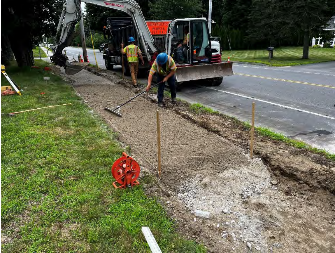
Photo 5 – Excavator operator placing Type A gravel with bucket, other crew member fine grading with rake.
