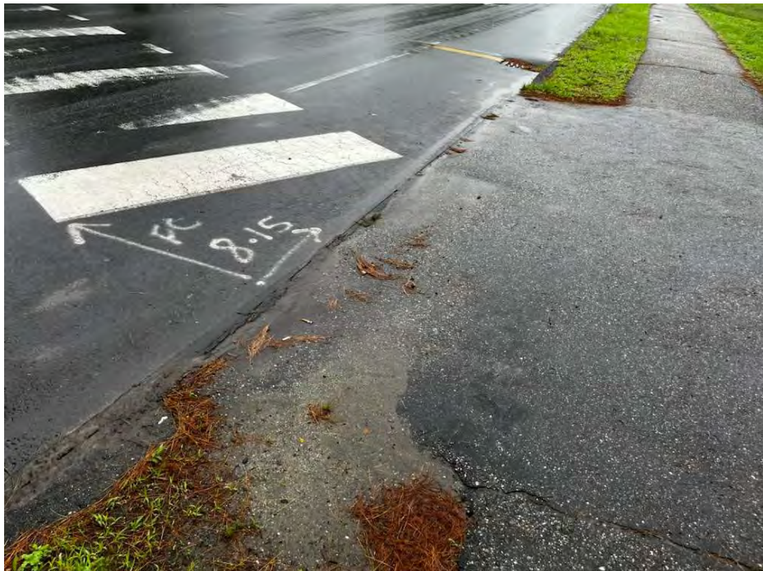
Photo 2 – Saw cut at gutter line of driveway apron at 385 Main Street.
