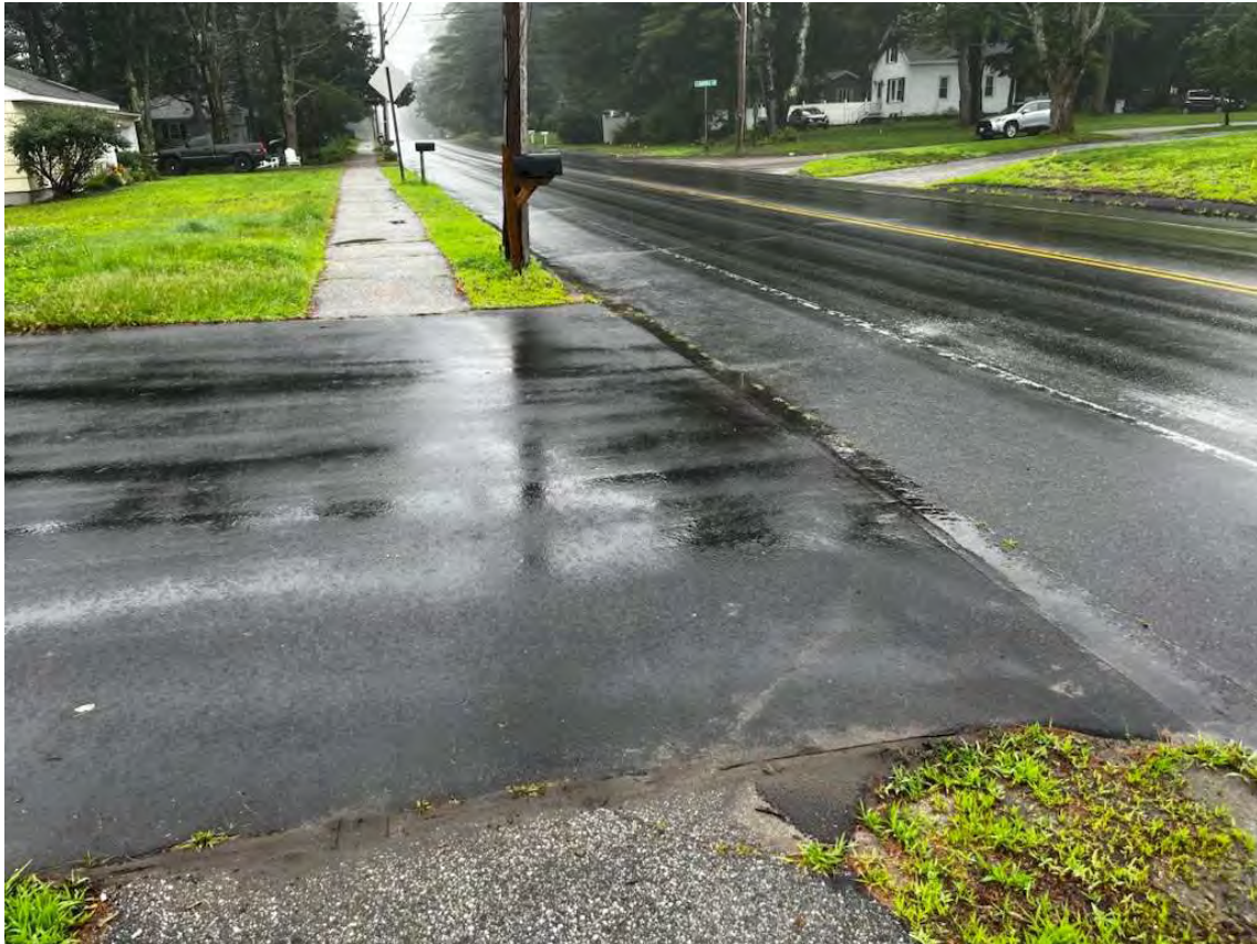
Photo 3 – Driveway apron at 387 Main Street protected (saw cut at sidewalk joint only).
