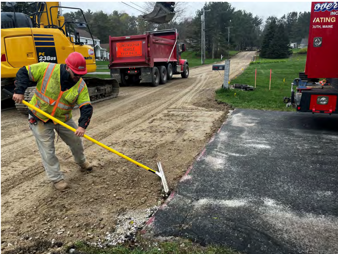
Photo 4 – Alex Grover surfacing the driveway aprons with material consistent with MaineDOT 703.06 Type A.
