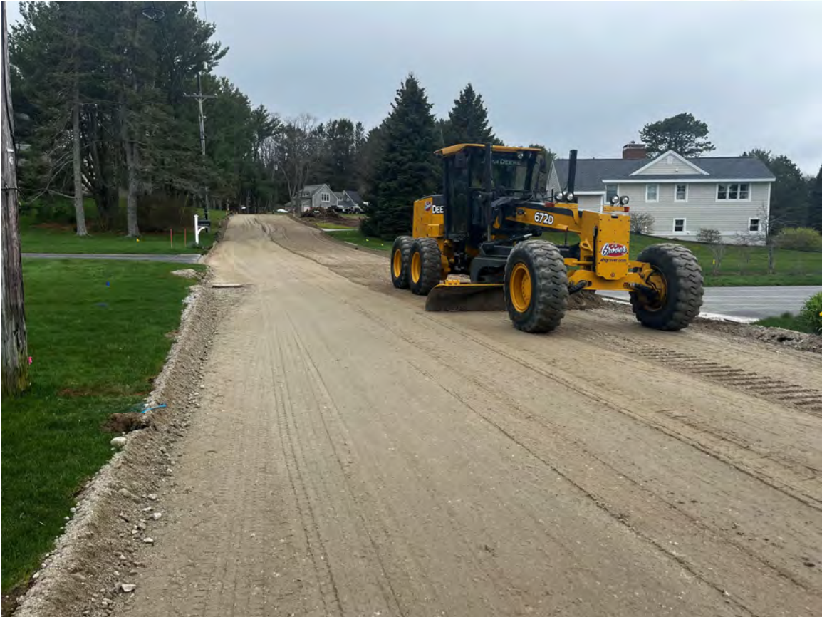
Photo 3 – Ben Grover operating the John Deere grader at an apparent 2% pitch towards the gutter.
