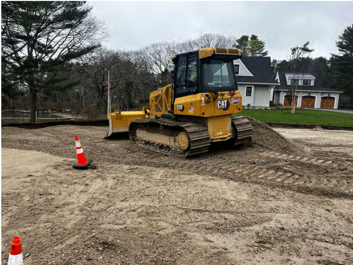
Photo 2 – Ben Grover operating dozer to push surface gravels into place.
