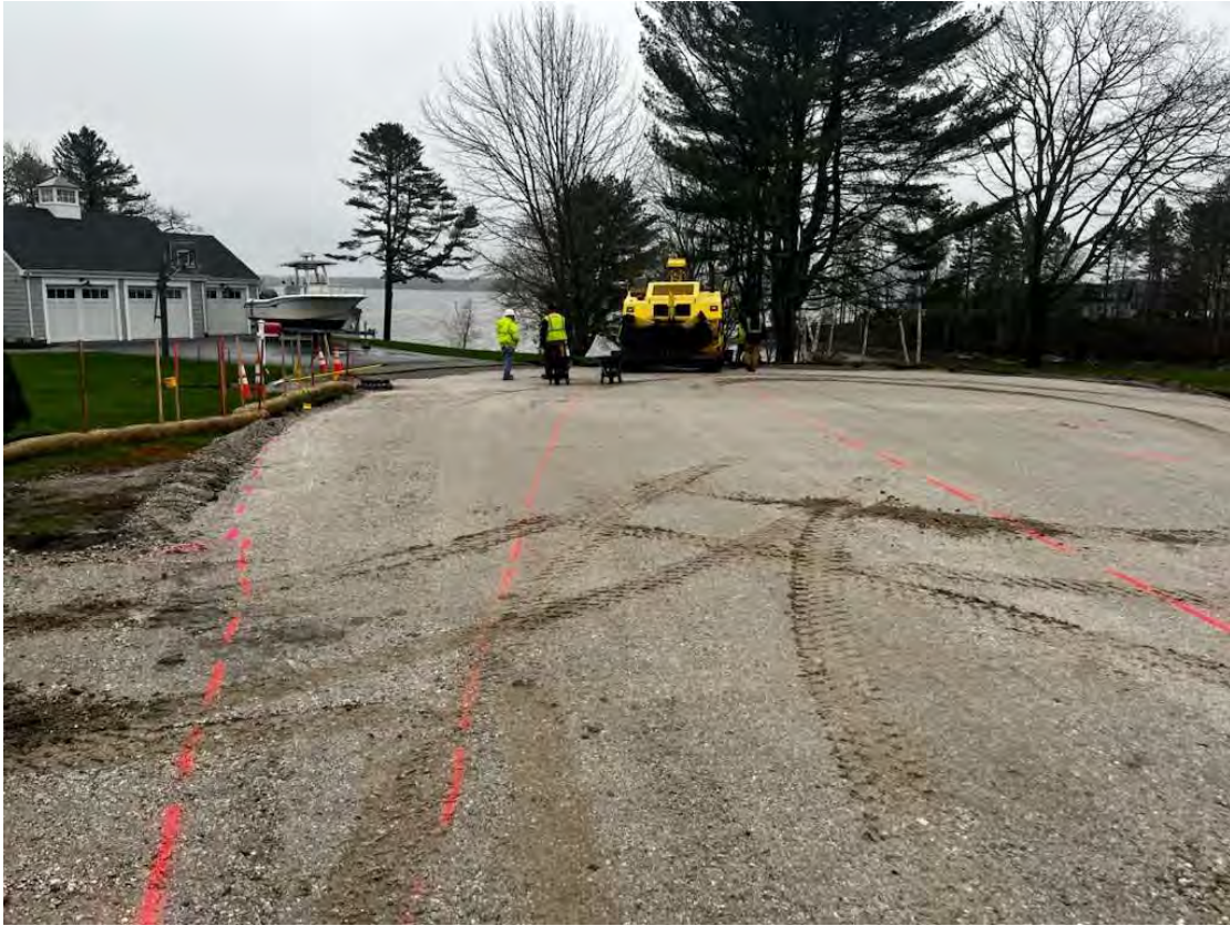
Photos 1 – Cul-de-sac area fine graded and compacted upon arrival.
