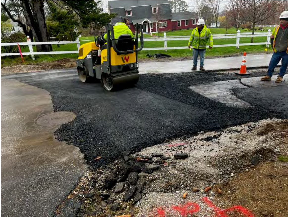
Photo 7 – Temporary patch of HMA placed between CB 9 and CB 10 for ease of vehicle traffic.
