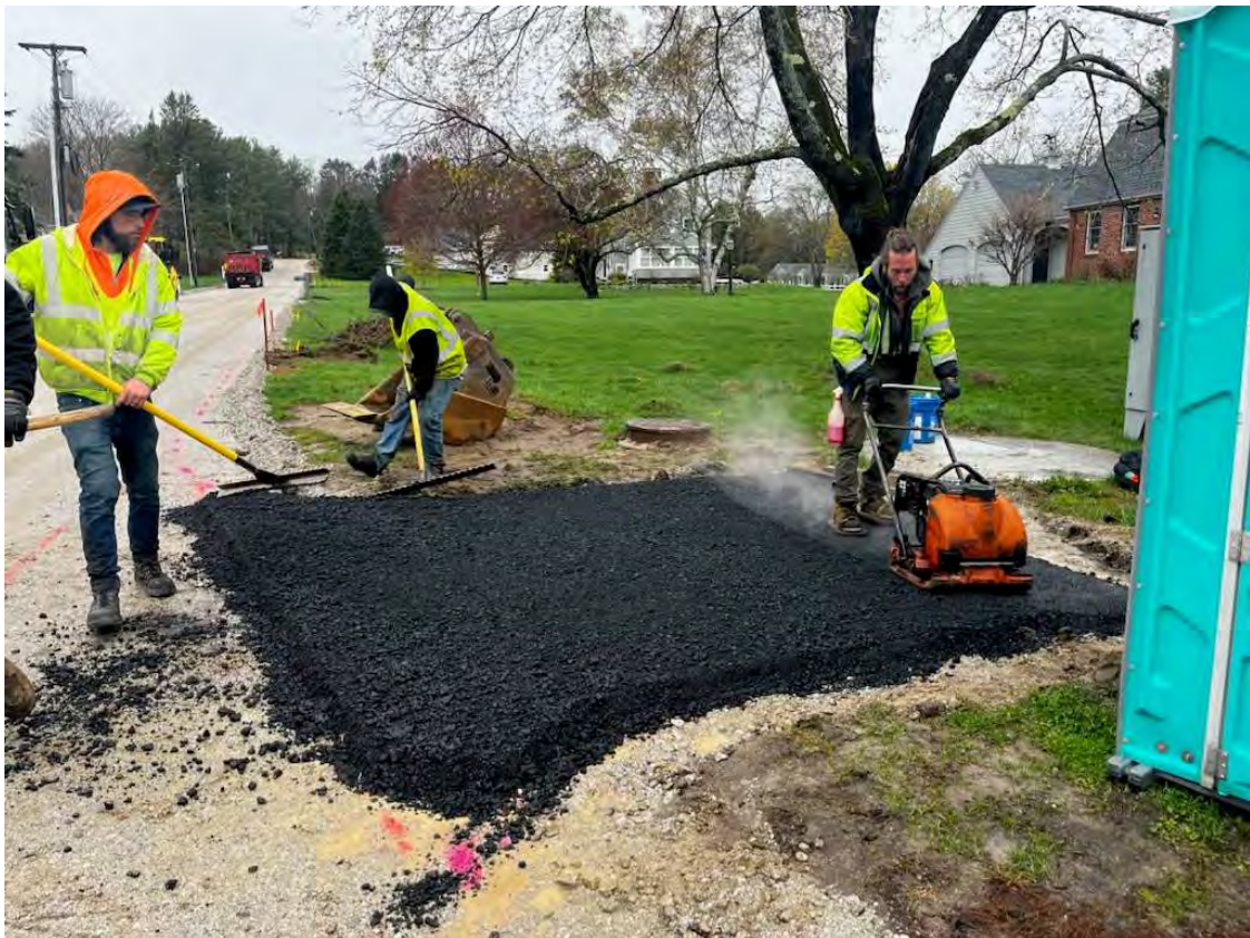
Photo 2 – Dayton Sand and Gravel crew compacting pad to pump station area.
