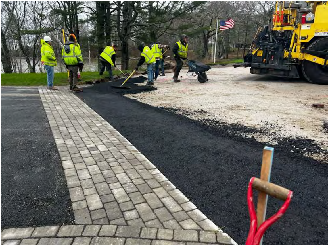
Photo 5 – Crew installing driveway apron by hand.
