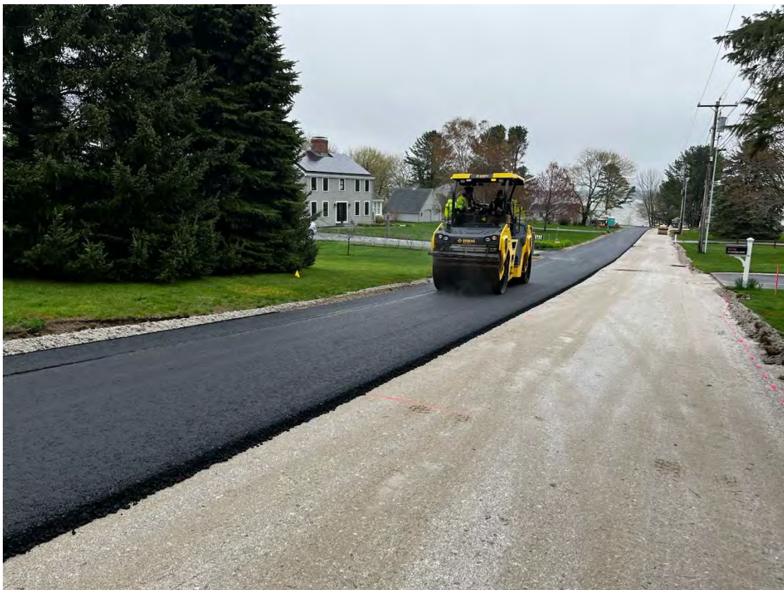
Photo 4 – 10-ton roller used to compact 19.0mm HMA.
