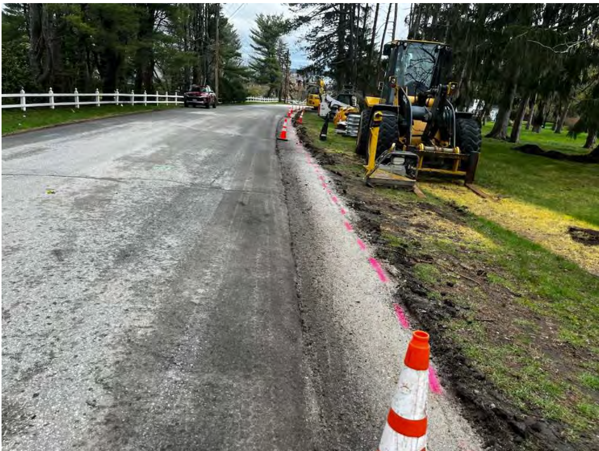
Photo 8 – Road widening/ Curb installation box cut area from STA 0+35 to STA 3+86.
