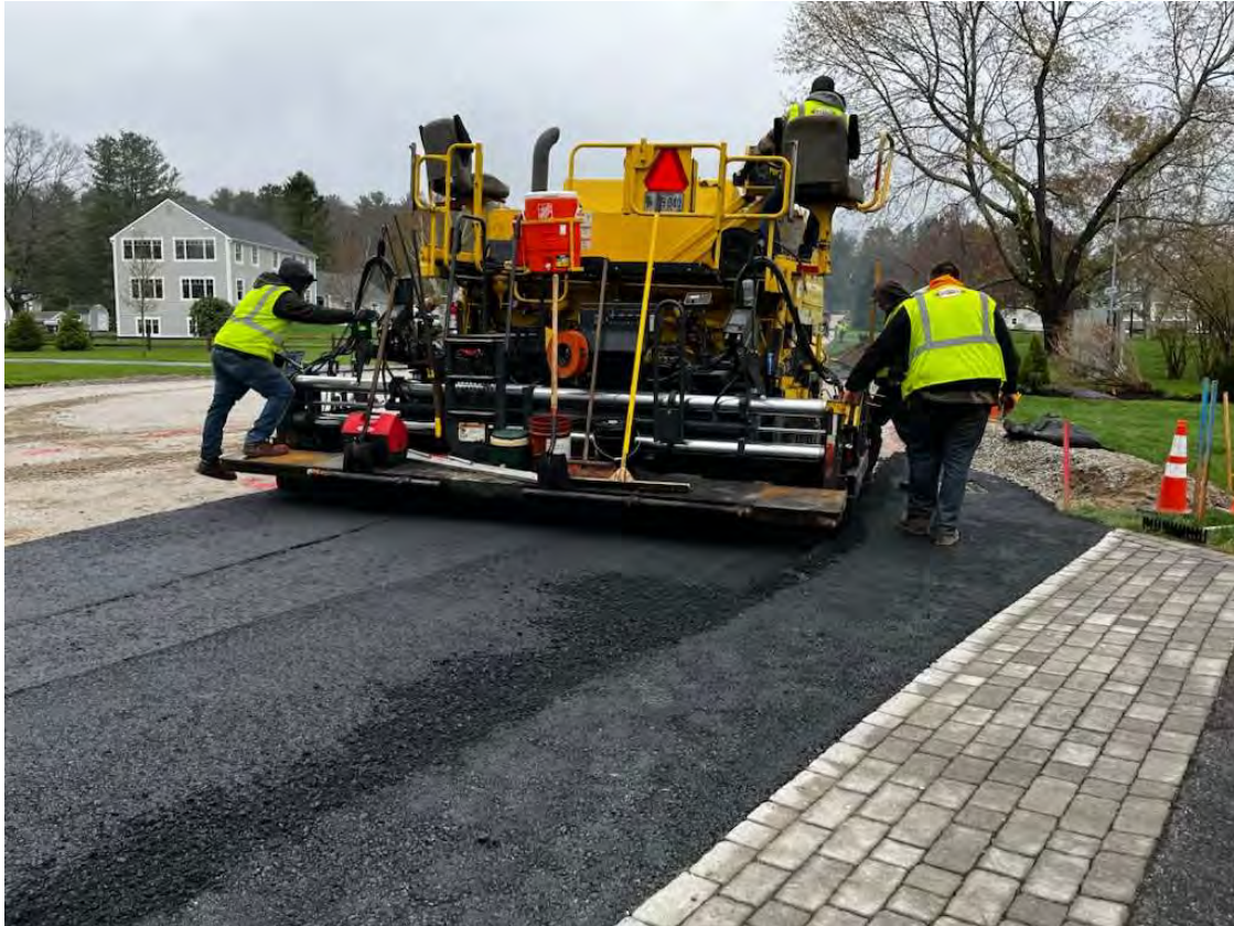
Photo 3 – Crew using a CR552 – Bomag paver to place pavement.
