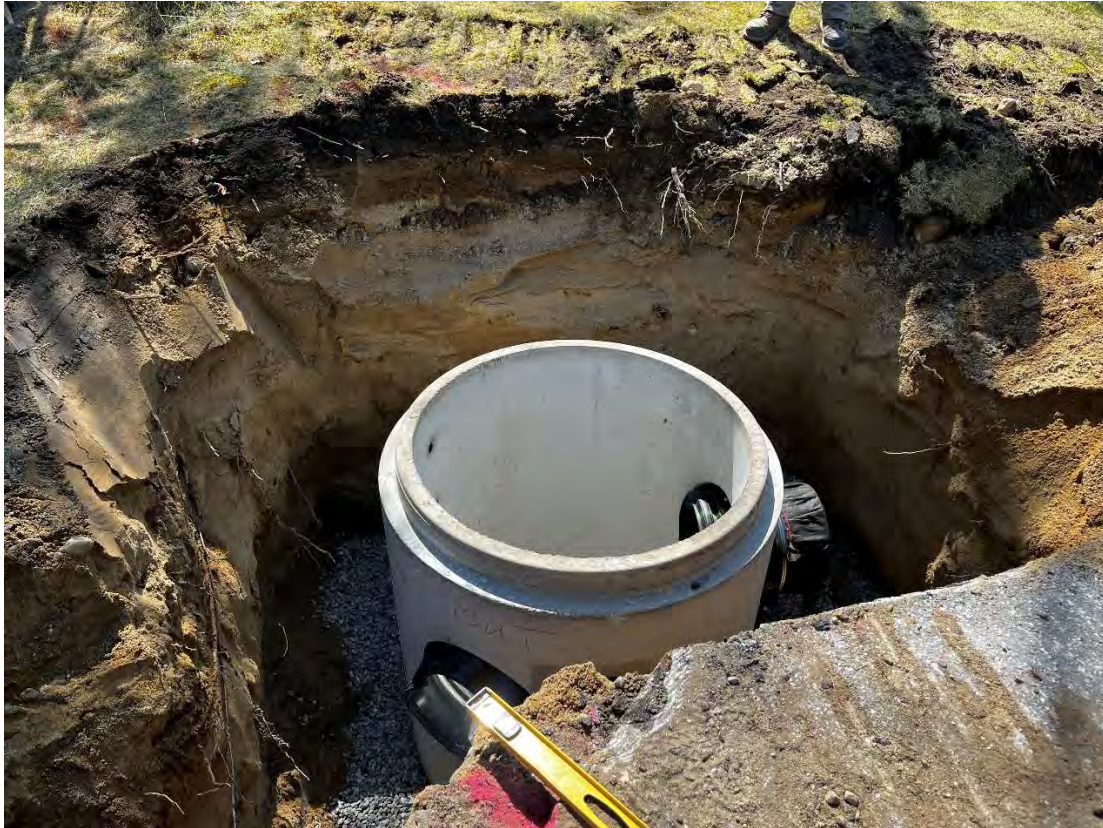
Photo 5 – CB 6 installed on a \frac{3}{4} " crushed stone base.
