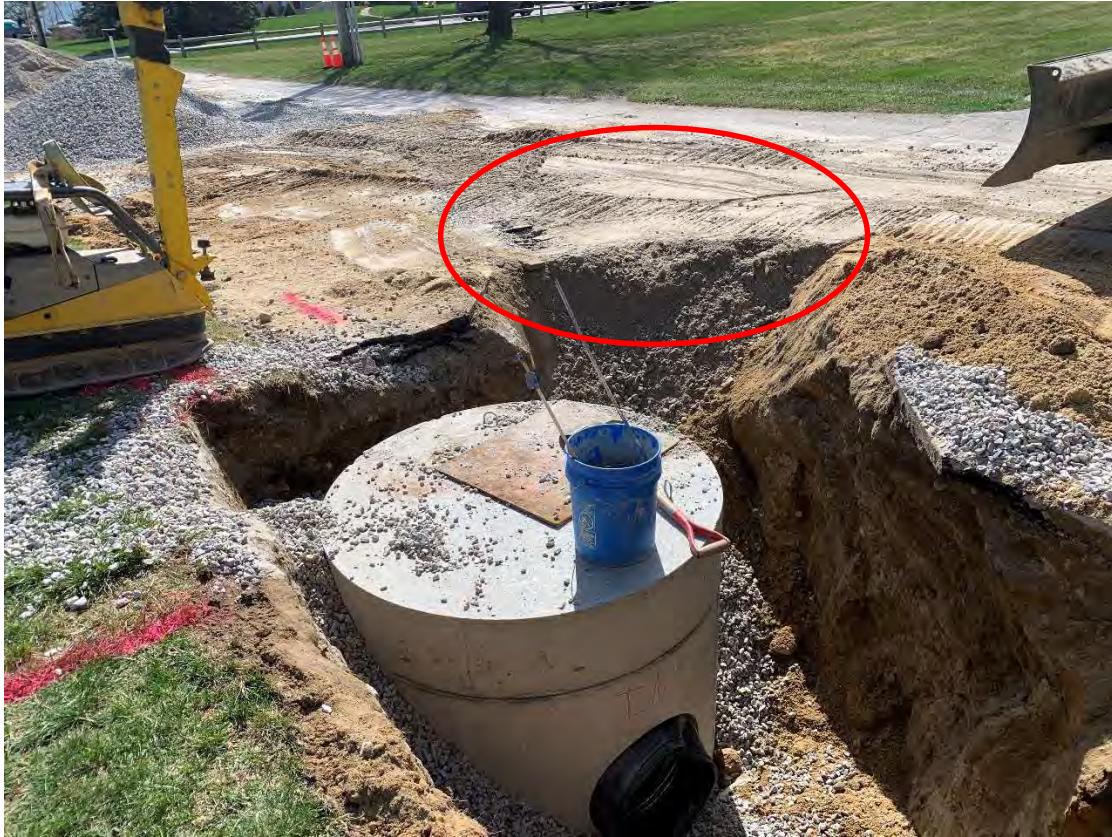
Photo 1 – Circled area is where DMH 3 has been backfilled until frame and cover can be installed.
