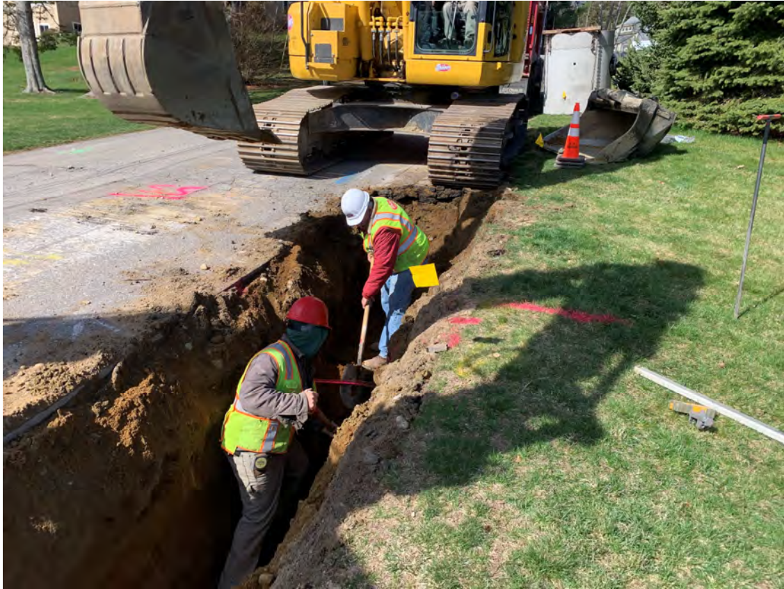
Photo 7 – Stewart and Crew member hand shoveling around underground utility.
