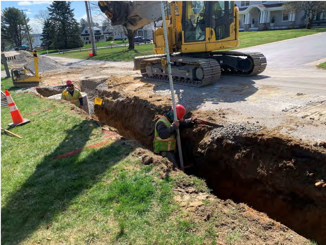
Photo 3 – Crew member using survey rod and laser level to check grade prior to SD installation.
