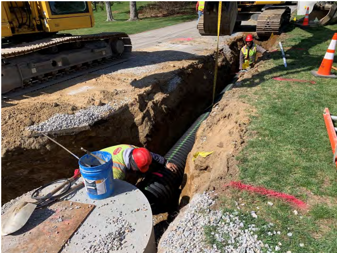
Photo 2 – 20-foot segment of 15" Perf. SD installed to CB 3.
