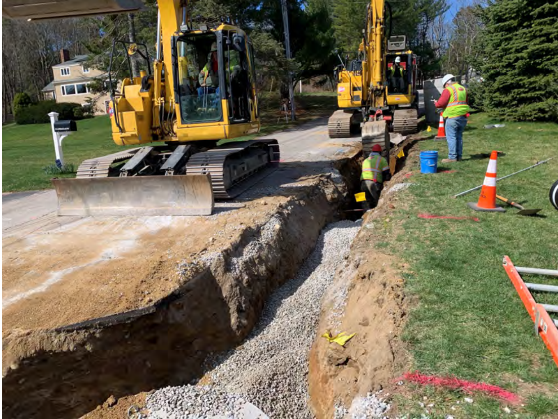
Photo 5 – MaineDOT 703.22 Type C \frac{3}{4} " Crushed stone placed approximately 1.75 feet above the spring line.
