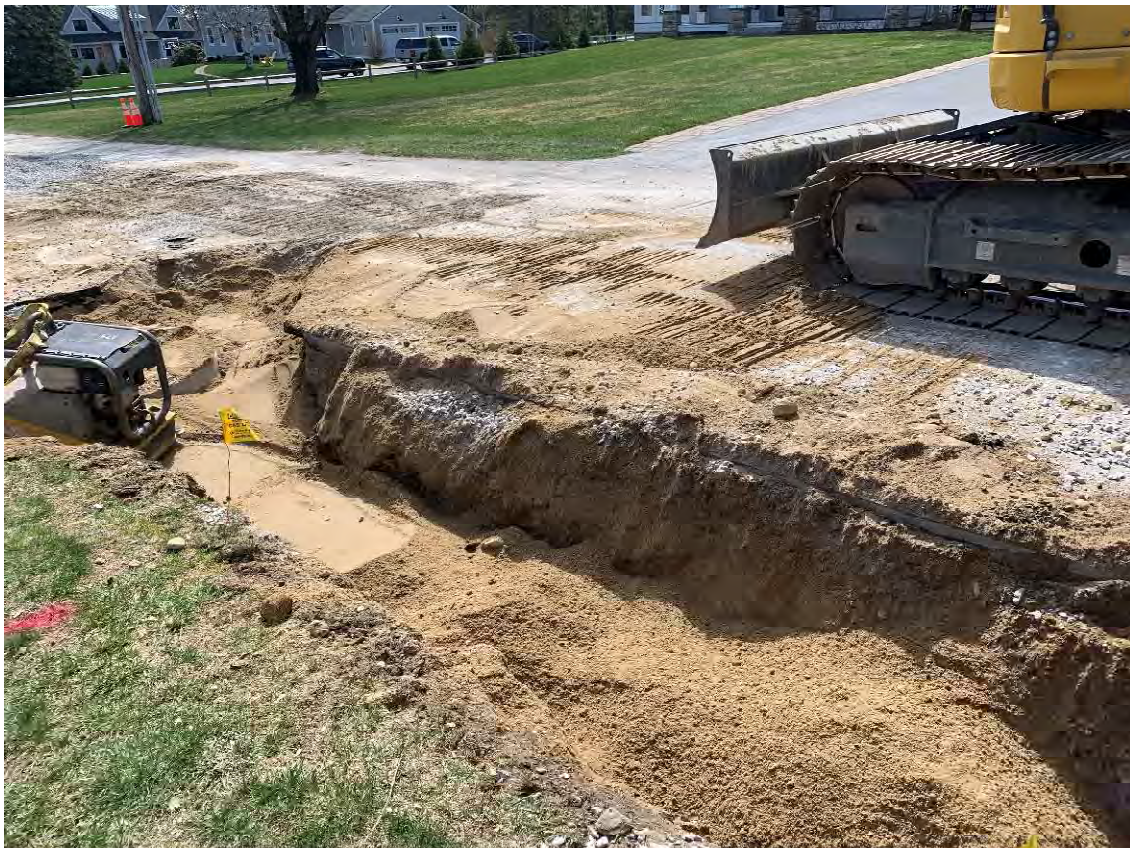
Photo 4 – CB 3 after it was backfilled with material consistent with MaineDOT 703.22 Type B Underdrain, also shown is a plate compactor compacting around the catch basin.
