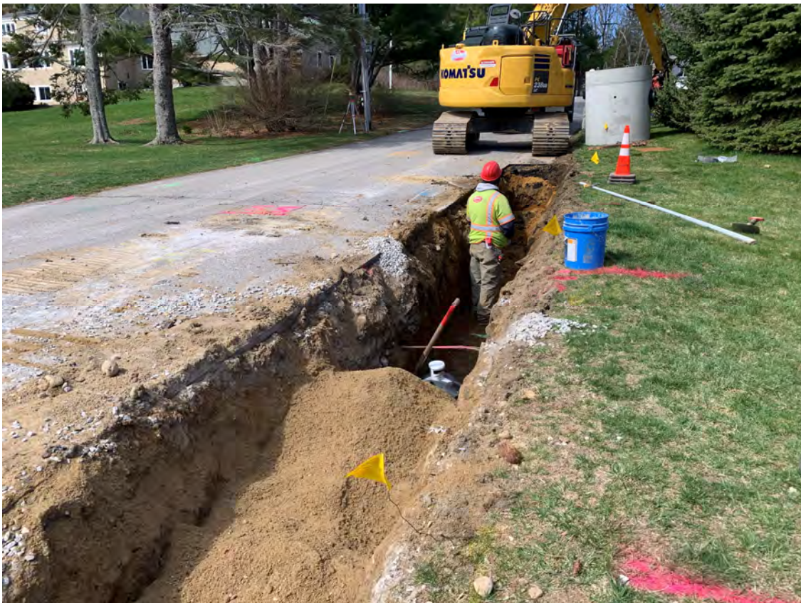
Photo 6 – MaineDOT 703.22 Type B underdrain placed in the trench to the subbase layer.
