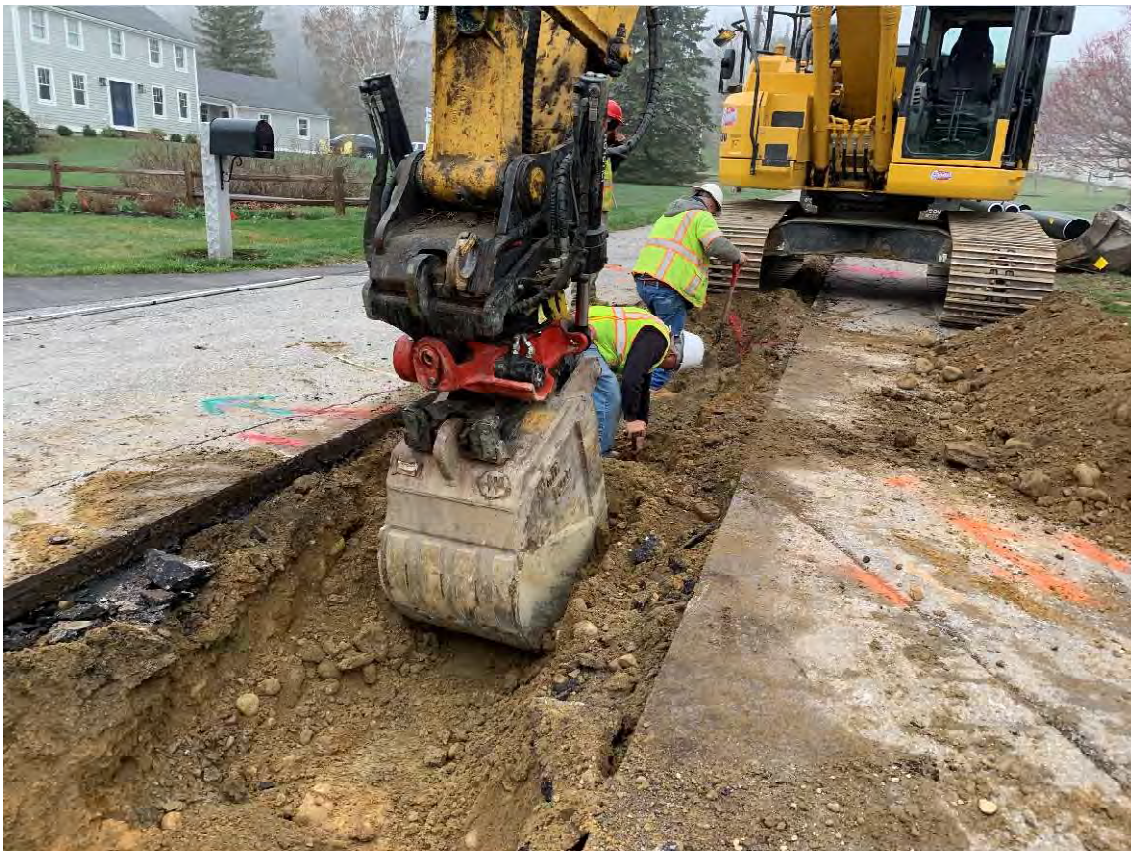
Photo 6 – Ben Grover and Stewart hand shoveling to locate underground utilities.
