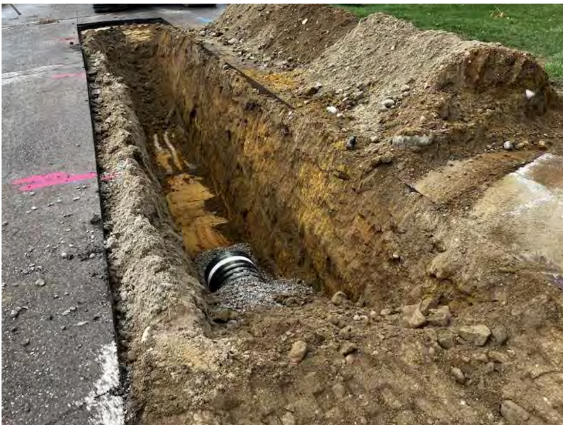
Photo 2 – Trench excavated full depth and no ledge rock present.
