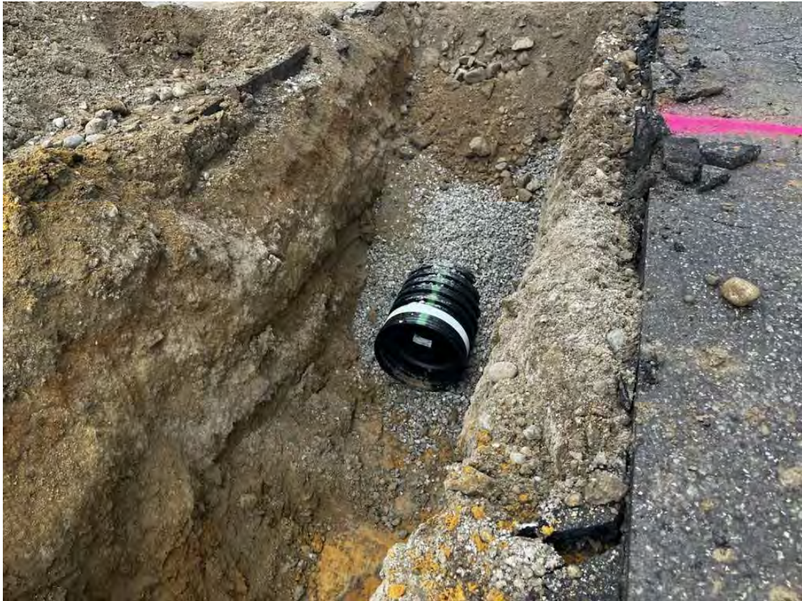
Photo 3 – Stormdrain embedded with \frac{3}{4} " stone and backfilled with suitable excavated material.
