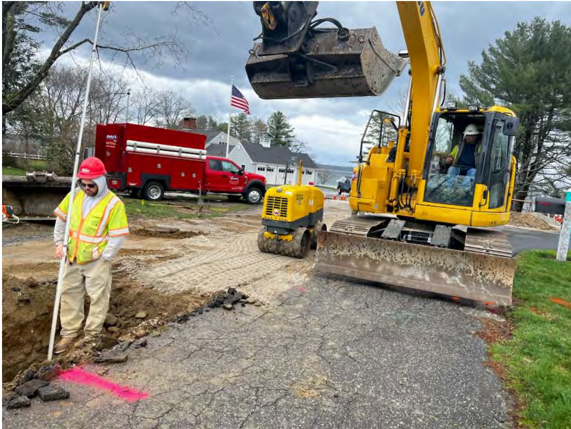
Photo 5 – Crew member using survey rod to check grade of pipe installed in trench.
