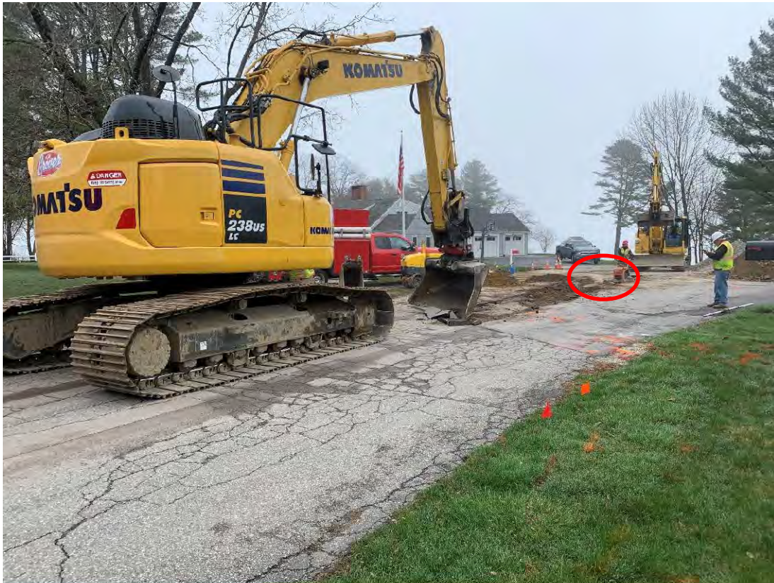
Photo 1 – DMH 1 (circled in red) installed. Matt Grover excavating towards DMH 2 for SD installation.
