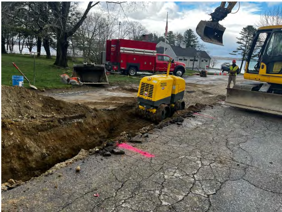
Photo 4 – Remote-Control Wacker Neuson compacting backfill material in the trench.
