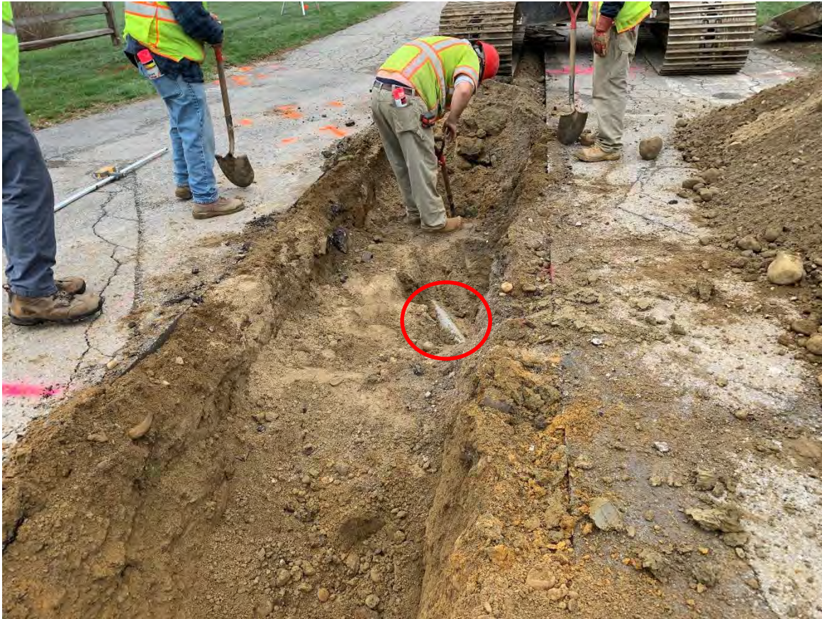
Photo 7 – Underground utility (circled in red) found and avoided.
