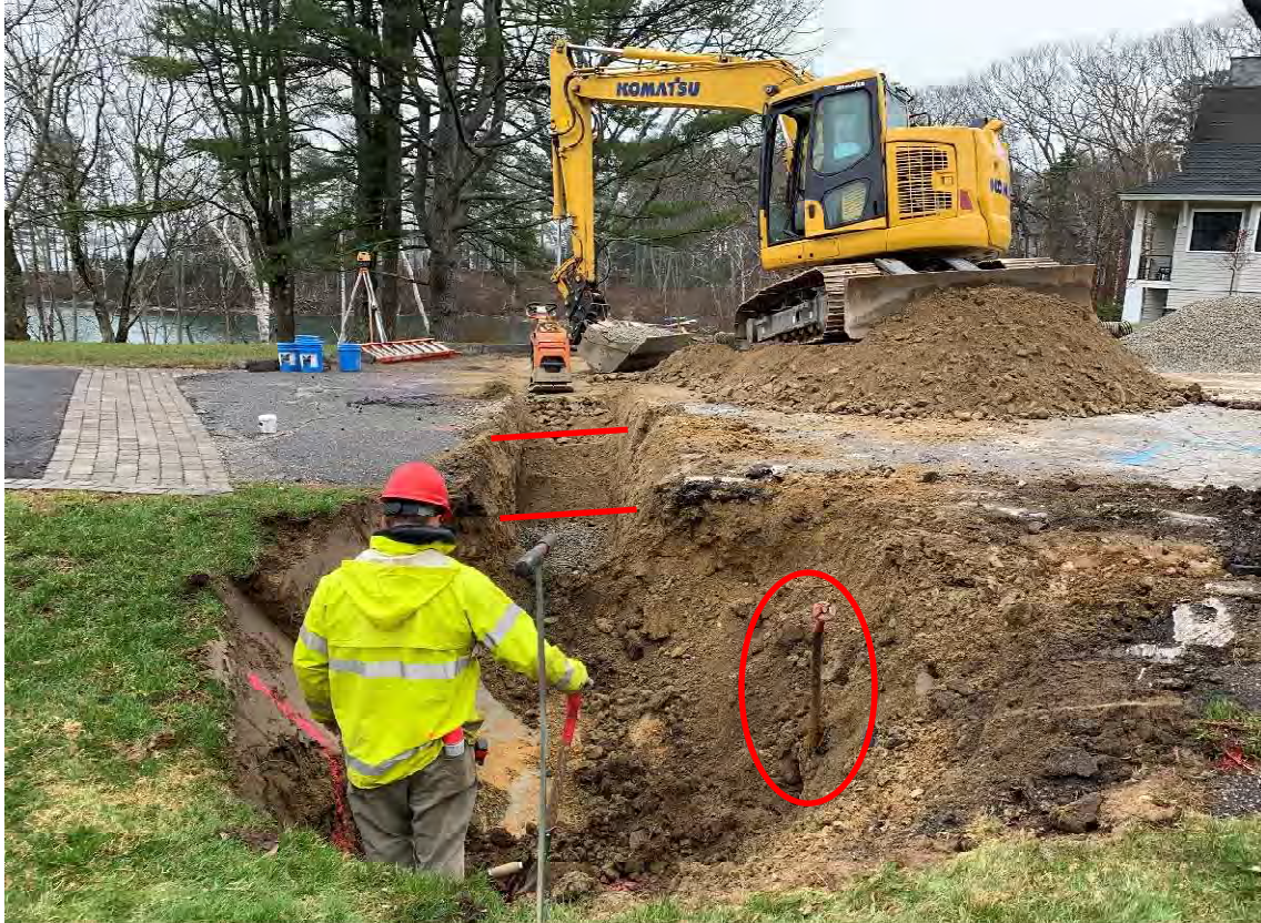
Photo 5 – The layers of gravel, separated by red lines are shown accordingly. Also, circled in red is a utility service avoided.
