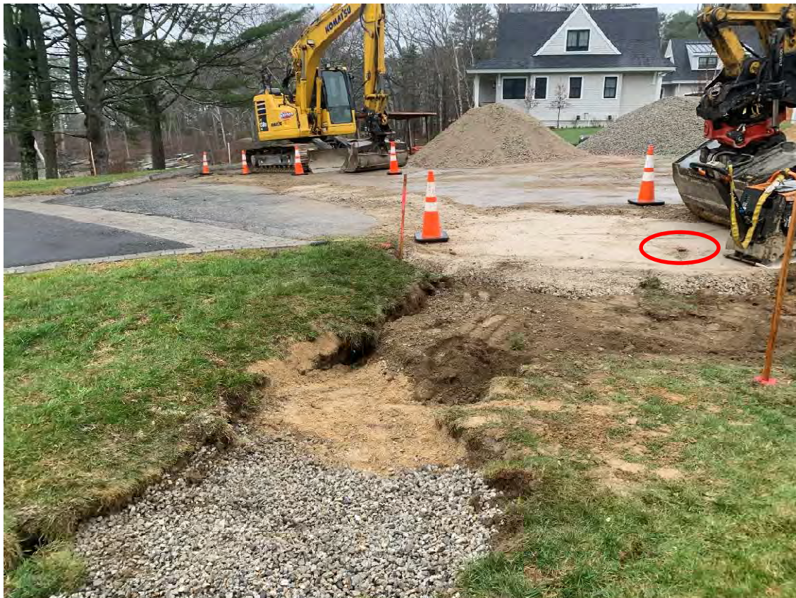
Photo 6 – CB 11 and CB 14 installed and temporary backfilled until frame and covers are installed. Circled in red is the same utility service circled in photo 5 backfilled accordingly.
