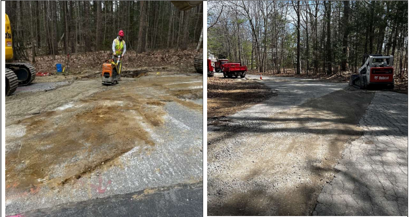
Photos 1 & 2 – Comparison pictures of before and after road sweeping around the same area. The left picture shows sediment onto the roadway from trench construction. The right side is post sweeping and water truck, sediment from the trenches do not appear to be on the roadway.
