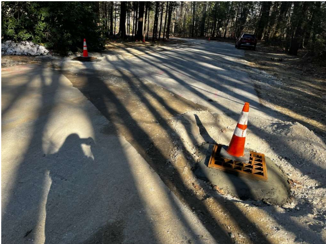
Photo 3 – Frame and covers installed on CBs # 20 and #21.
