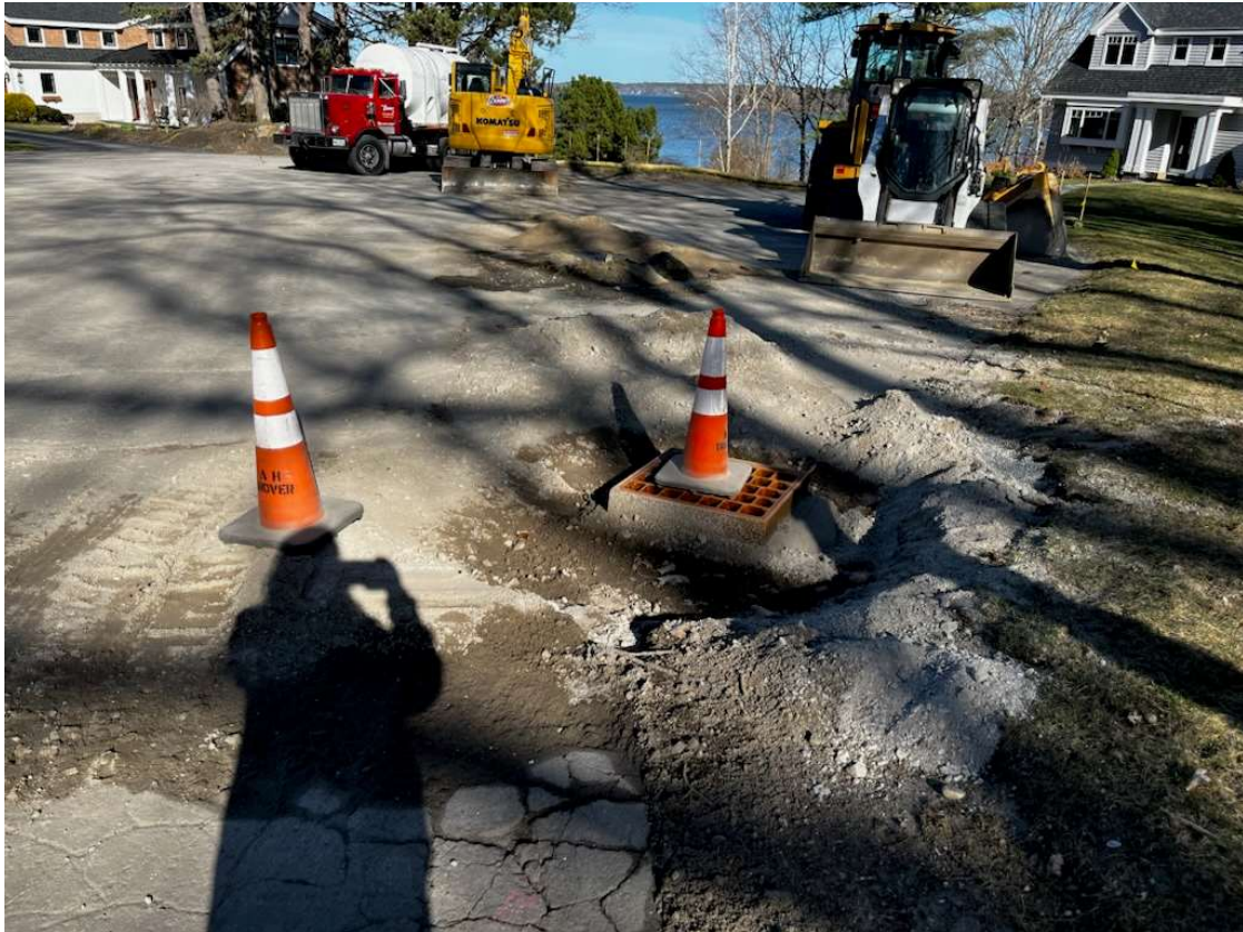
Photo 4 – Frame and cover installed on CB #26. Water truck used is also pictured in the background.
