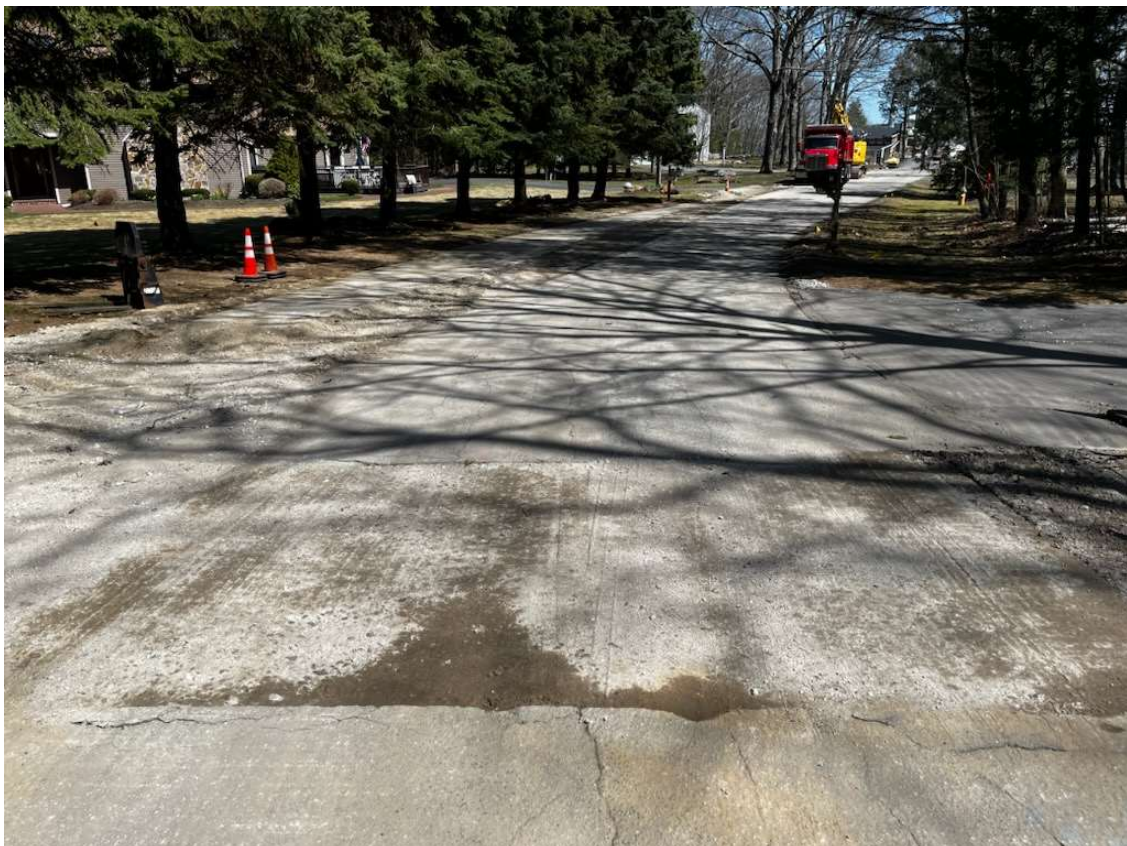
Photo 5 – Cross trench area (between CB #24 & CB #25) fine graded for paving.
