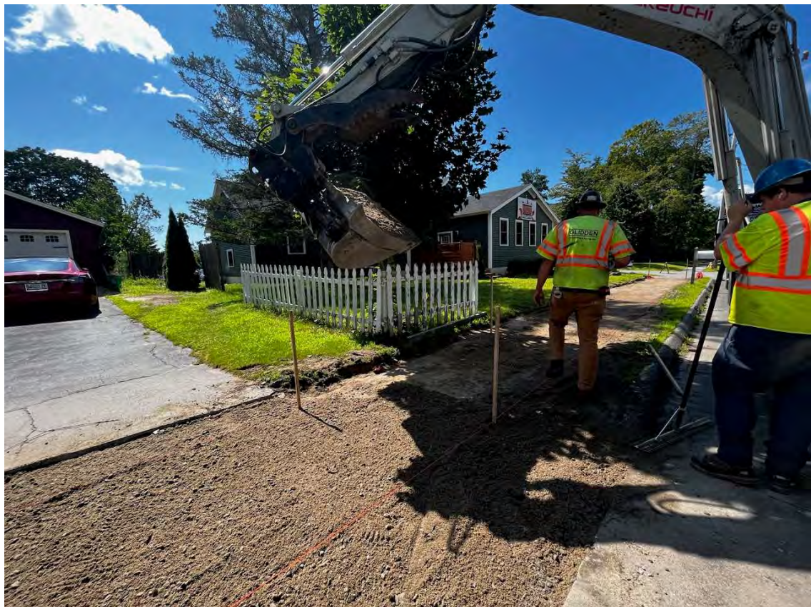
Photo 2 – Base gravel installed by excavator between sidewalk limits.
