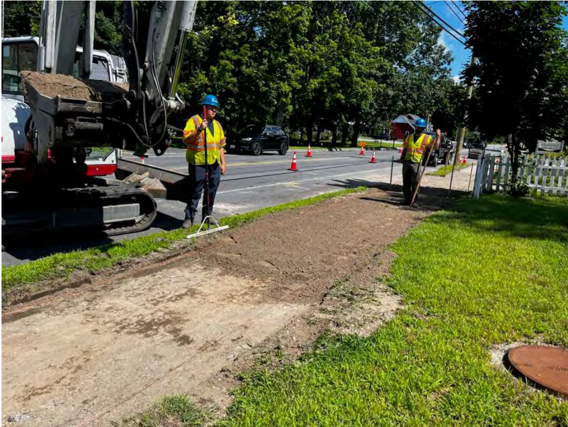
Photo 3 – Crew using rake to fine grade base gravels prior to compaction.
