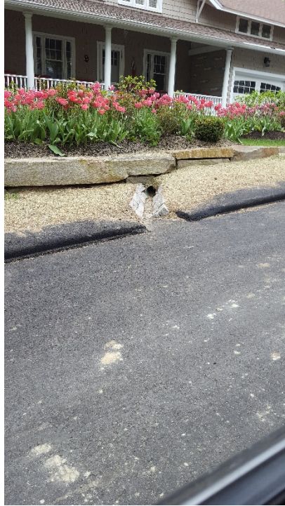
Pavers installed as outlet protection at #25 Birch Lane
