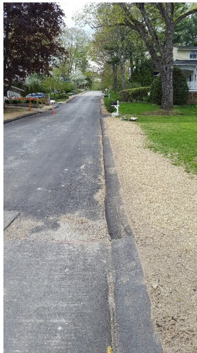
Fill, Loam, Seed, and Mulch installed to back up curb on Birch Lane
