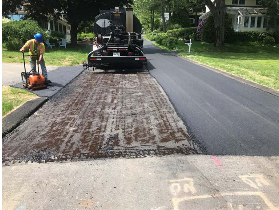
Photo 1 – Tack placed on Birch Lane prior to 9.5mm HMA.
