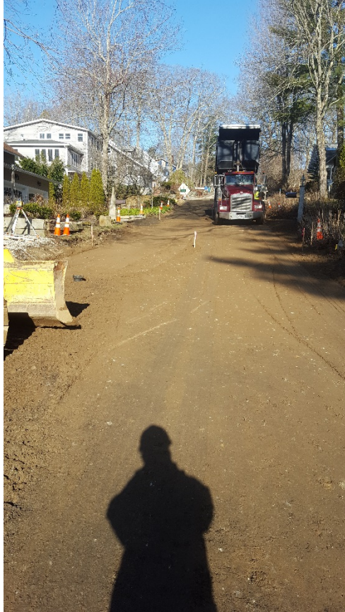
Placing of base gravel, looking west
