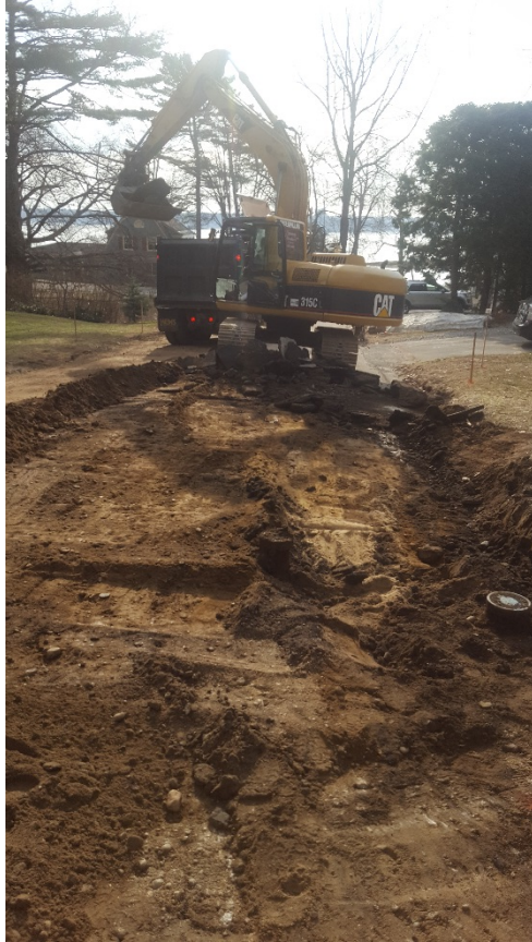
Box cutting the roadway, looking east
