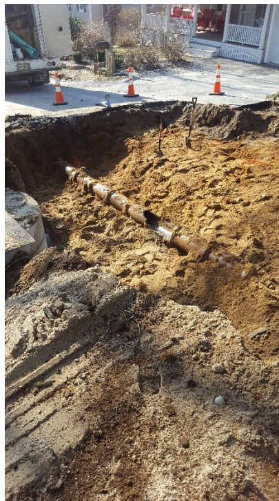
Pipe uncovered between the two proposed catch basins.
