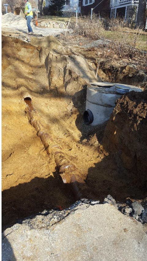
Pipe uncovered between the two proposed catch basins.
