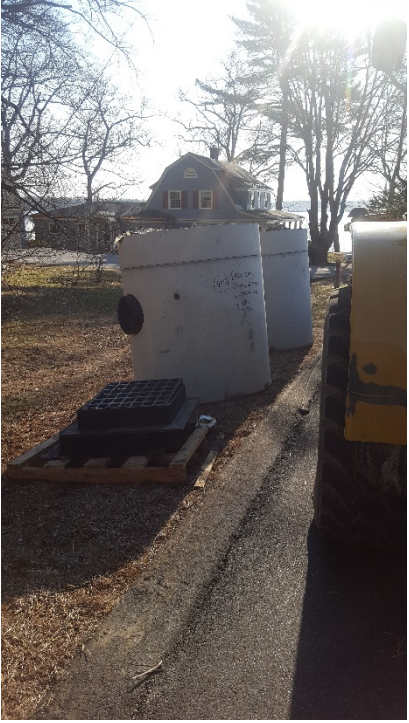
Catch basins and frames delivered to the site.
