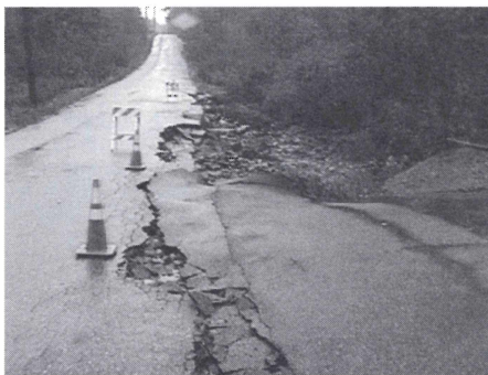
Examples of the October Storms and the damage caused: Powell Road Culvert and Harris Road Washout
