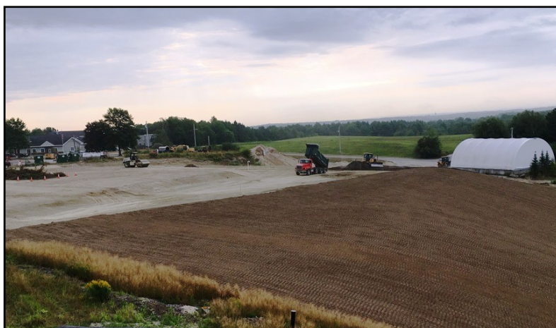
Capping the old "stump dump" and regrading the area.
