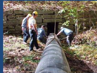
Blanchard Road Culvert Lining 2001 by Highway Department
